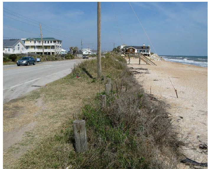
Shore erosion threatens State Road A1A.
