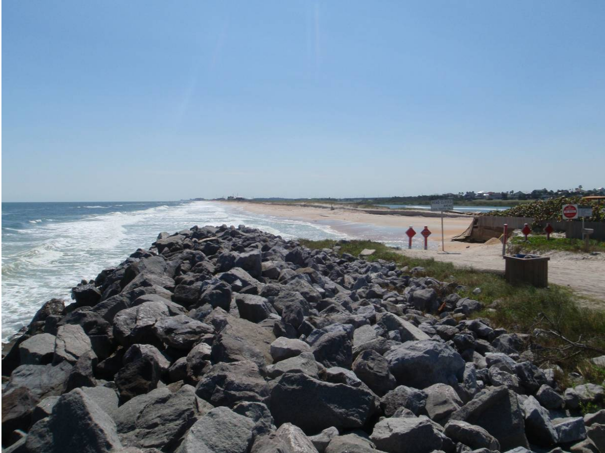
Figure 2-7. Looking south along the Summer Haven reach (around R198). Granite revetment fronts the paved remnant of Old SR A1A. The breach at R200 is shown in the middle of the picture, just beyond the “Road Closed” sign.
