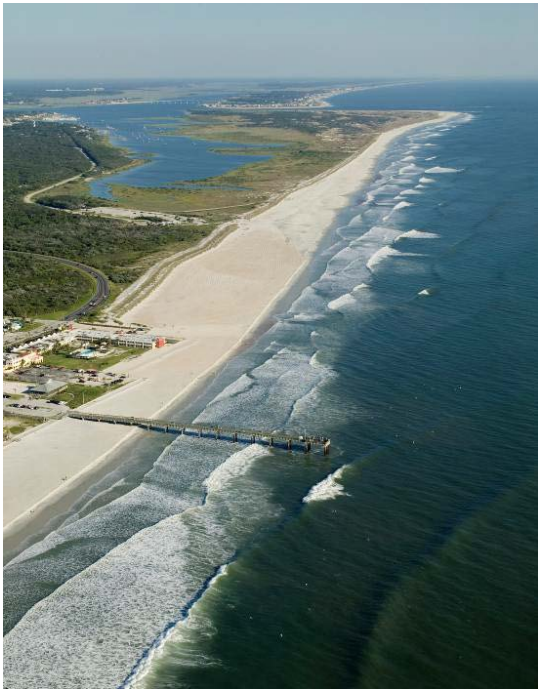
St. Augustine Beach – Constructed
