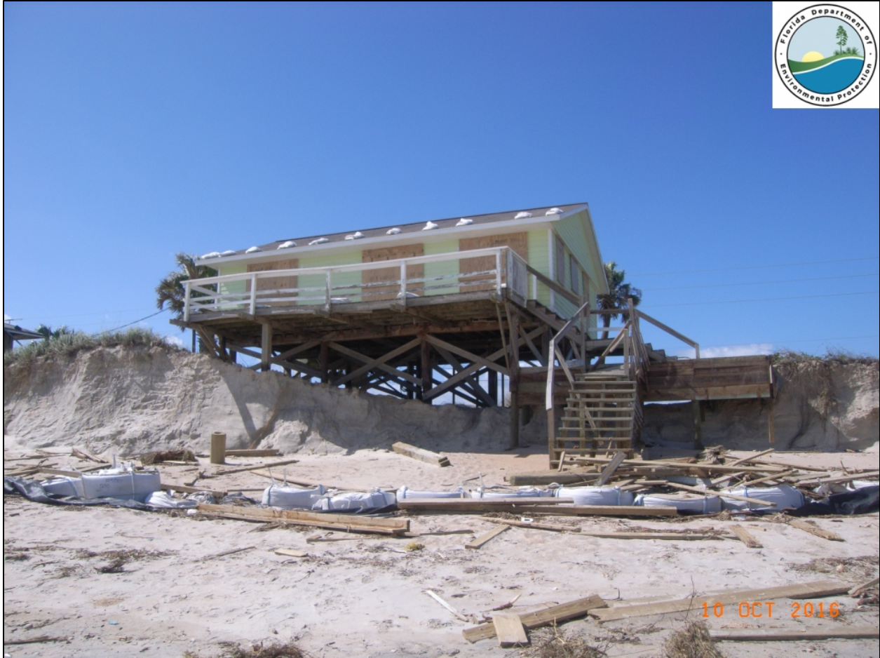
Figure 4-6. Hurricane Matthew damage in the vicinity of R116 on Oct. 10, 2016. Note debris from destroyed dune walkovers and other structures. Note dune scarping and erosion below house. Image courtesy of Florida Department of Environmental Protection.
