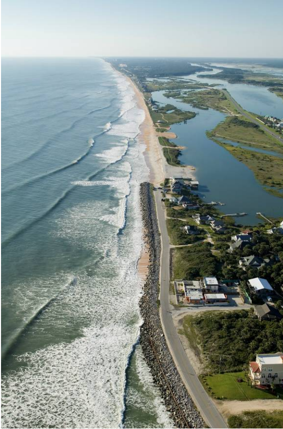
Figure 2-4. Summer Haven reach viewed from its northern end. Granite revetment protects paved sections of Old SR A1A.
