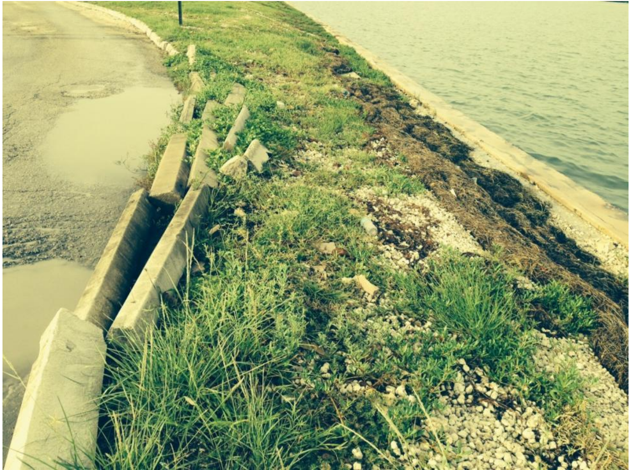
Figure 1-6: Inundation and waves breaking over the seawall carried seaweed behind the wall during an October 7, 2014 extreme high tide event. Ponding water indicates land subsidence under the road.
