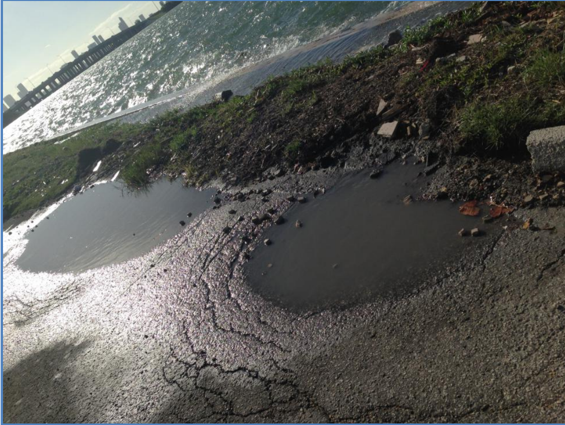
Figure 1-4: Segment of seawall showing waves overtopping wall and land subsidence causing potholes along perimeter road landward of seawall.
