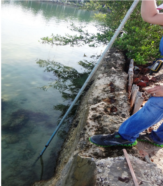
Figure 2-1: Northern segment of existing seawall.
