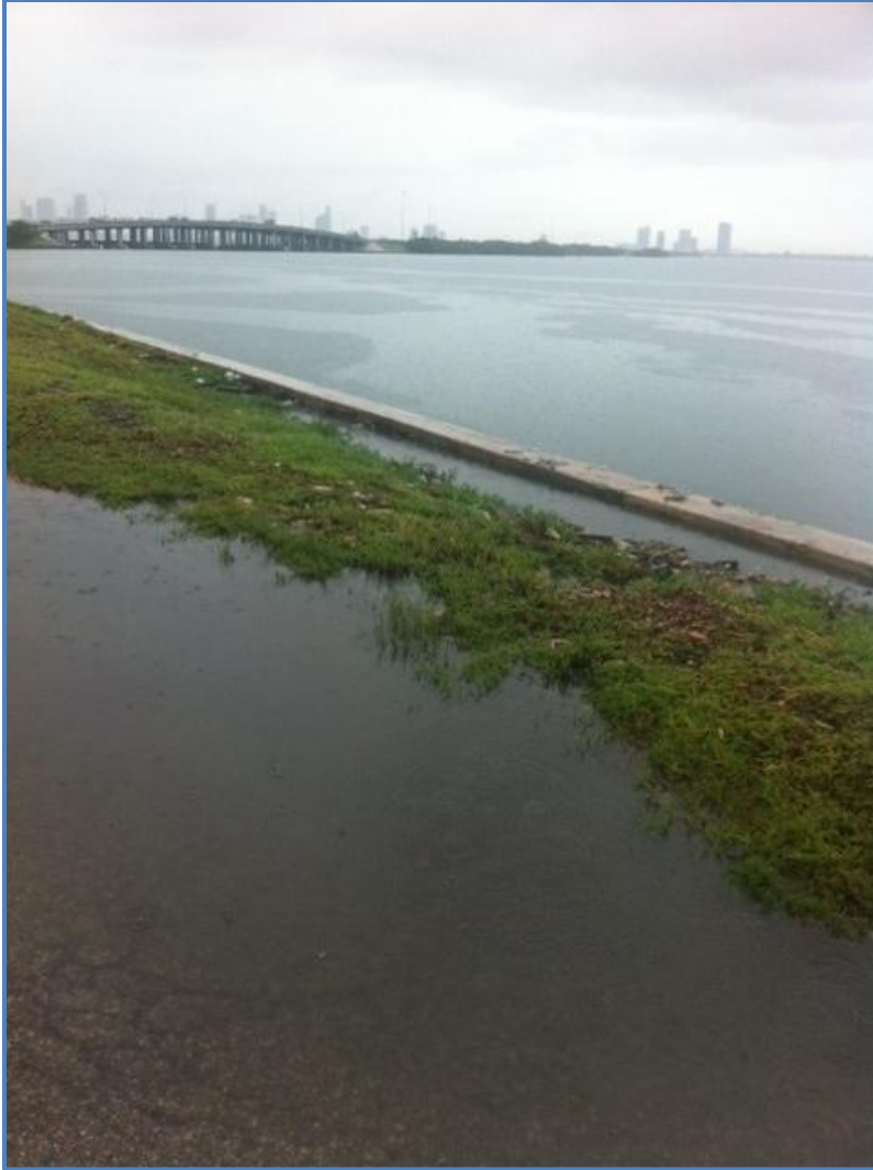
Figure 1-3: Biscayne Bay elevated to the top of the seawall during a July 2013 extreme high tide event. Standing water behind the wall, covering the perimeter road, resulted from overtopping of the seawall.
