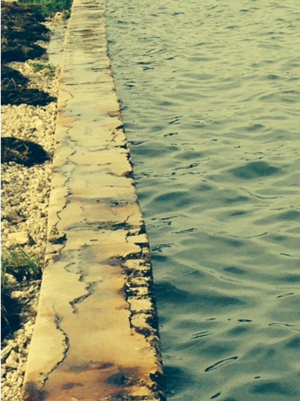
Figure 1-7: Rusting rebar and cracking throughout the seawall (2014).
