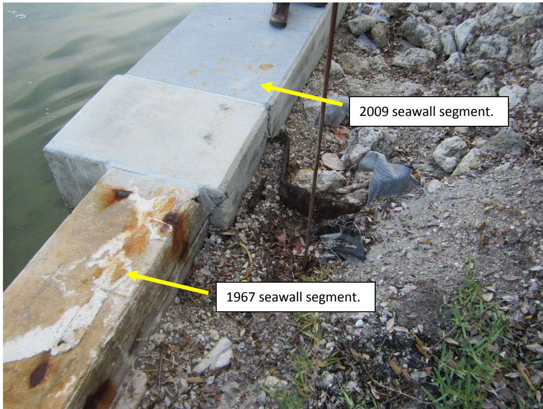
Figure 2-4: The newest segment of seawall; 130 feet constructed in 2009 and tying into the 1967 segment.
