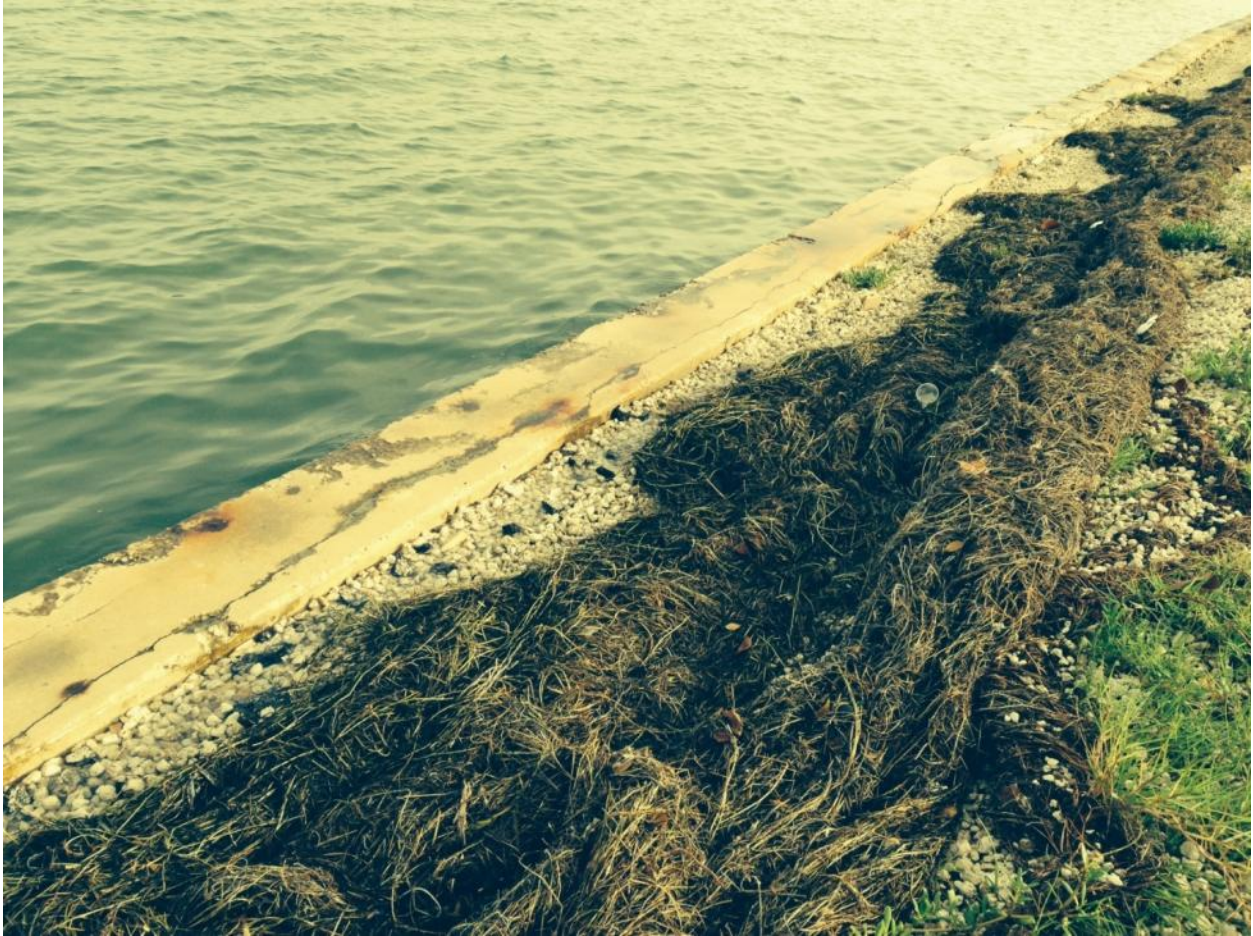
Figure 1-5: Inundation and waves breaking over the seawall carried seaweed behind the wall during an October 7, 2014 extreme high tide event.
