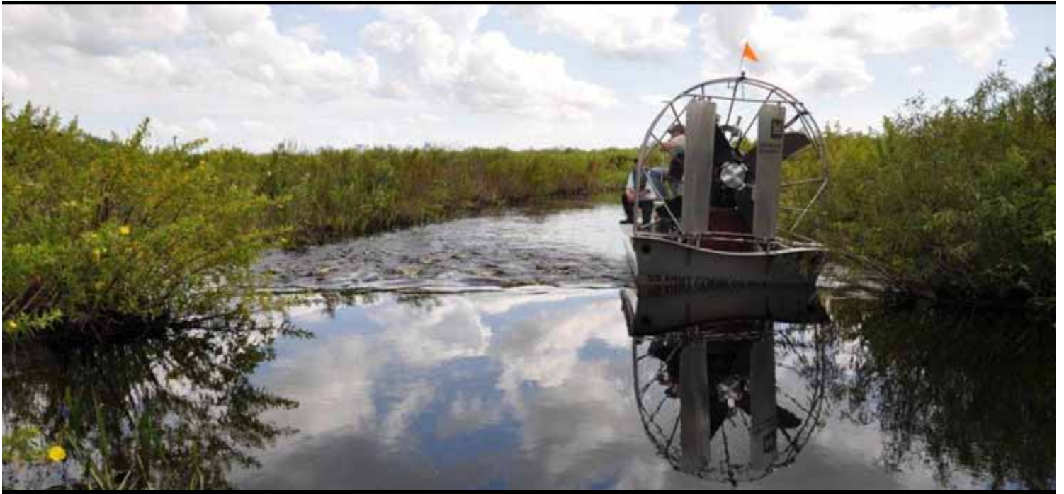
After inspecting the channel at Cowbone Marsh, Regulatory Division issued a cease and desist order, requiring the Florida Fish and Wildlife Commission to stop sidecasting dredged material into the channel. (PHOTO BY BY BRIAN CORNWELL)
