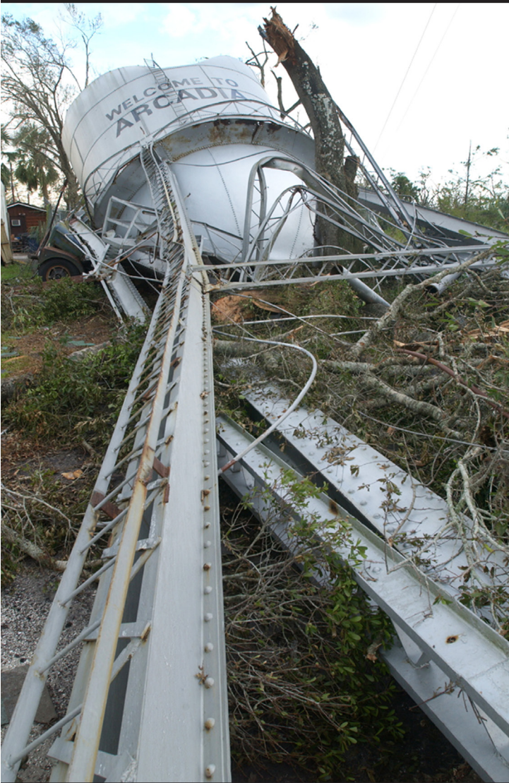
The water tower in Arcadia took a direct hit from the winds of Hurricane Charley after it roared ashore Aug. 13, 2004. The storm intensified greatly before making landfall, with winds increasing from 105 to 145 mph. (USACE file photo)
