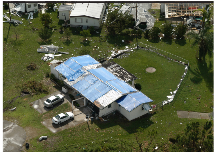
A home near Punta Gorda was outfitted with a temporary "Blue Roof" following Hurricane Charley. The Corps provided temporary roofing solutions for more than 115,000 structures following the 2004 storms. (USACE file photo)
