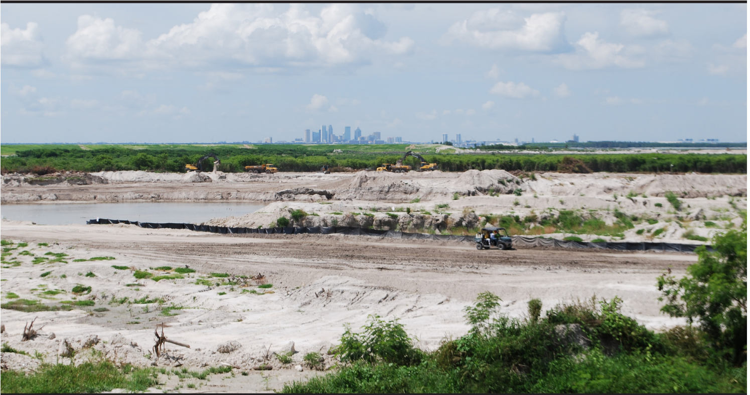
With Tampa in the distance, dike construction continues at 3-D to increase its capacity to 15-million cubic yards for use in disposing Tampa Harbor Project dredged materials.
