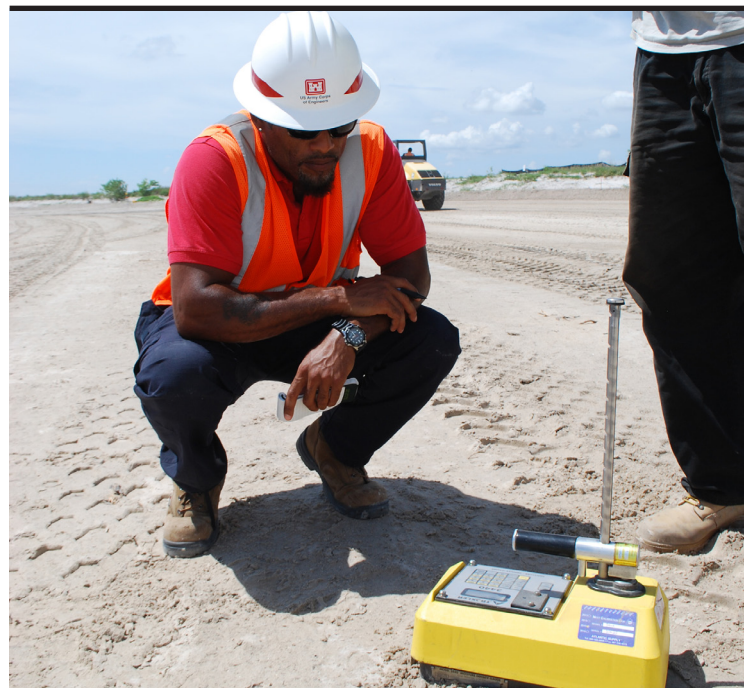
Corps Inspector Kenny Poindexter takes a soil compaction reading along new work on the dike.
