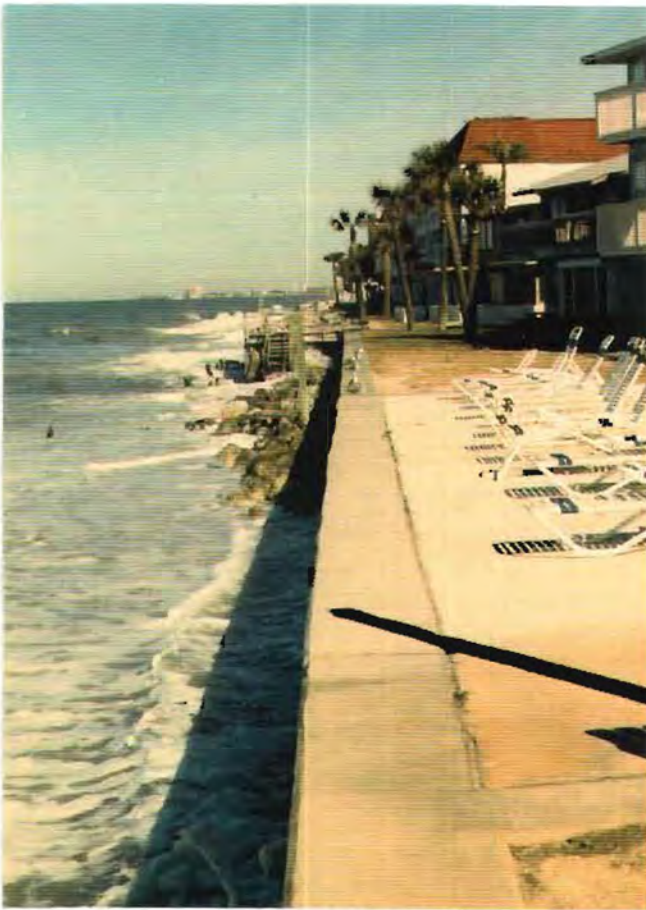
J-2 Shoreline View of Belleair Beach looking north from Morgan Drive city park during high tide period
