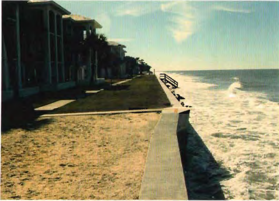
J-4 Shoreline View of Belleair Beach looking south from Morgan Drive city park during high tide period
