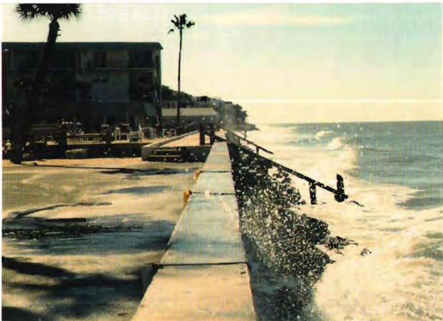
J-12 Shoreline View of Belleair Beach looking south from northern city limits during high tide period
