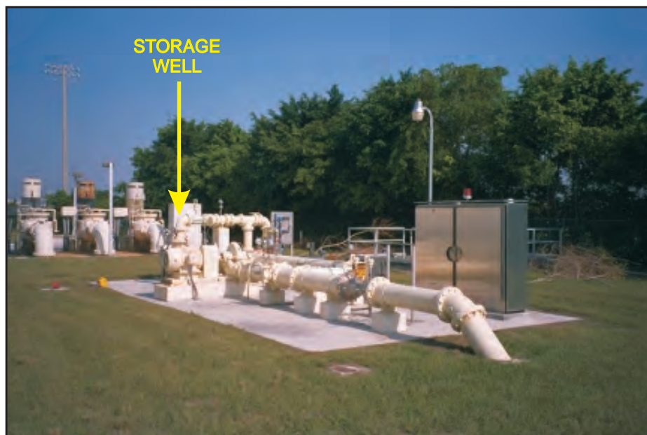
Figure 15. Wellhead piping, valves, and control system for the aquifer storage and recovery well at the Springtree Water Treatment Plant site in Broward County. Storage well on left side of concrete pad as shown by arrow.
