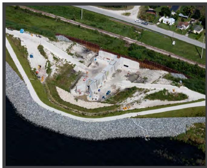
*Construction continues at the Herbert Hoover Dike on Water Control Structure S-272, the replacement for Culvert 13 located near Canal Point on the southeast side of Lake Okeechobee. S-272 is one of 21 culvert replacement projects that were under contract with Jacksonville District at the end of 2015. (USACE File photo)*
