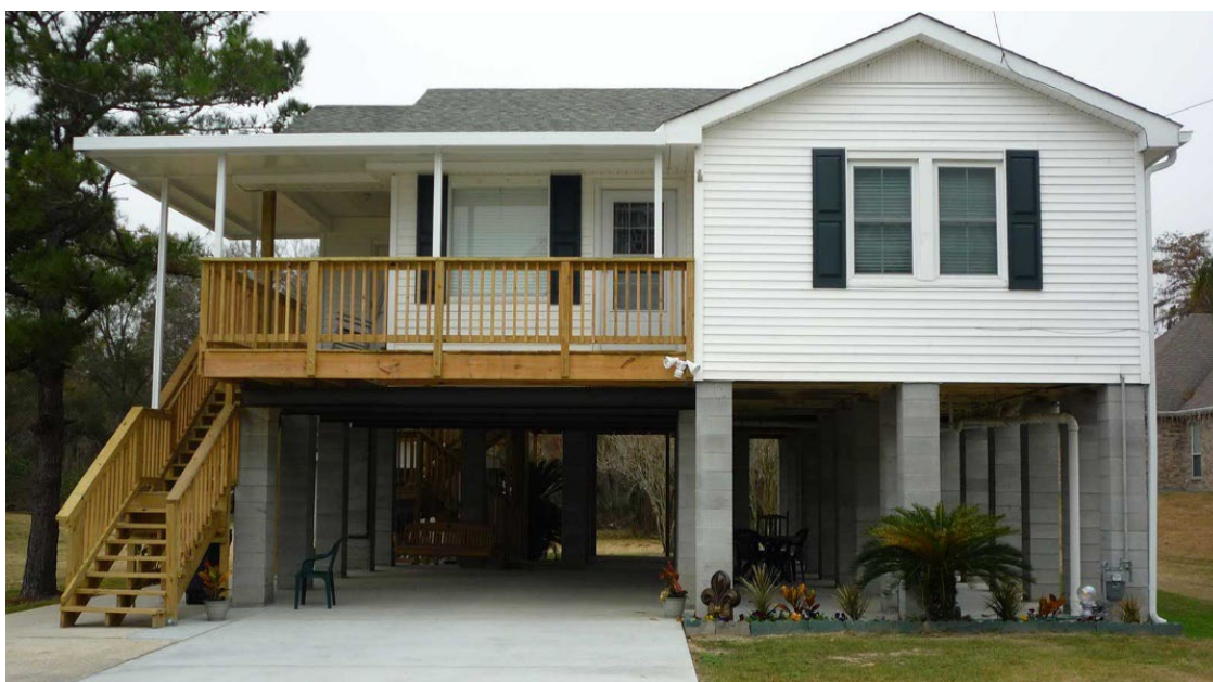
Figure 9-1. Elevated Home with Drive-Under Garage, New Orleans, Louisiana
