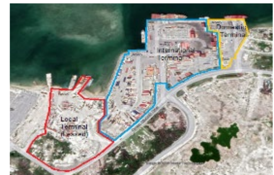
U.S. Northern Command Port Facility Assessment (Marsh Harbour, Bahamas)
