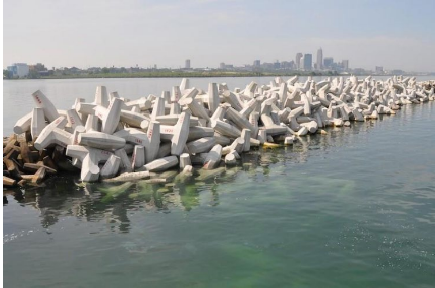
Figure 3: Concrete Armor Units (Dolosse) Implemented in Corps' Cleveland Harbor East Breakwater Project (2016)
