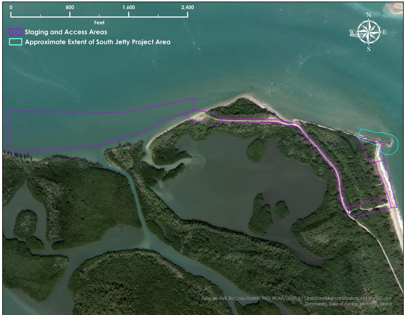
Figure 2: Close Up Overview of Project Area
