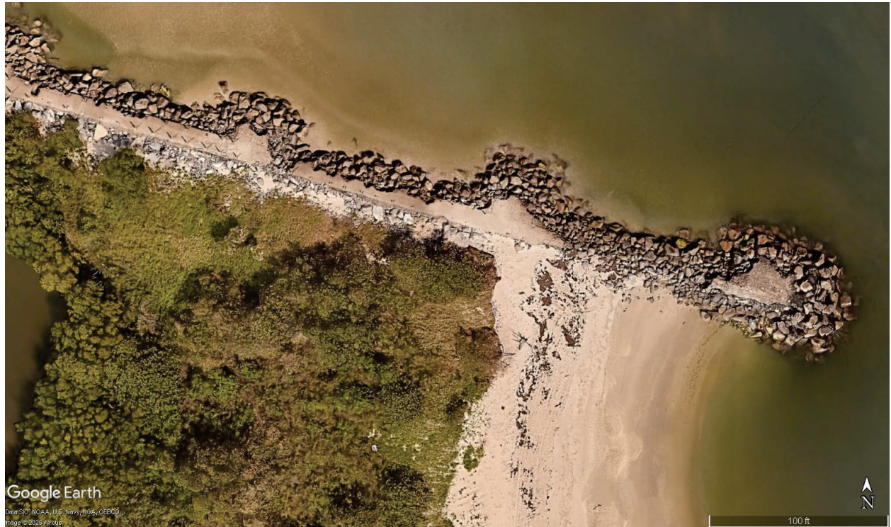
Figure 2: Close up view of the St. Lucie South Jetty Head
