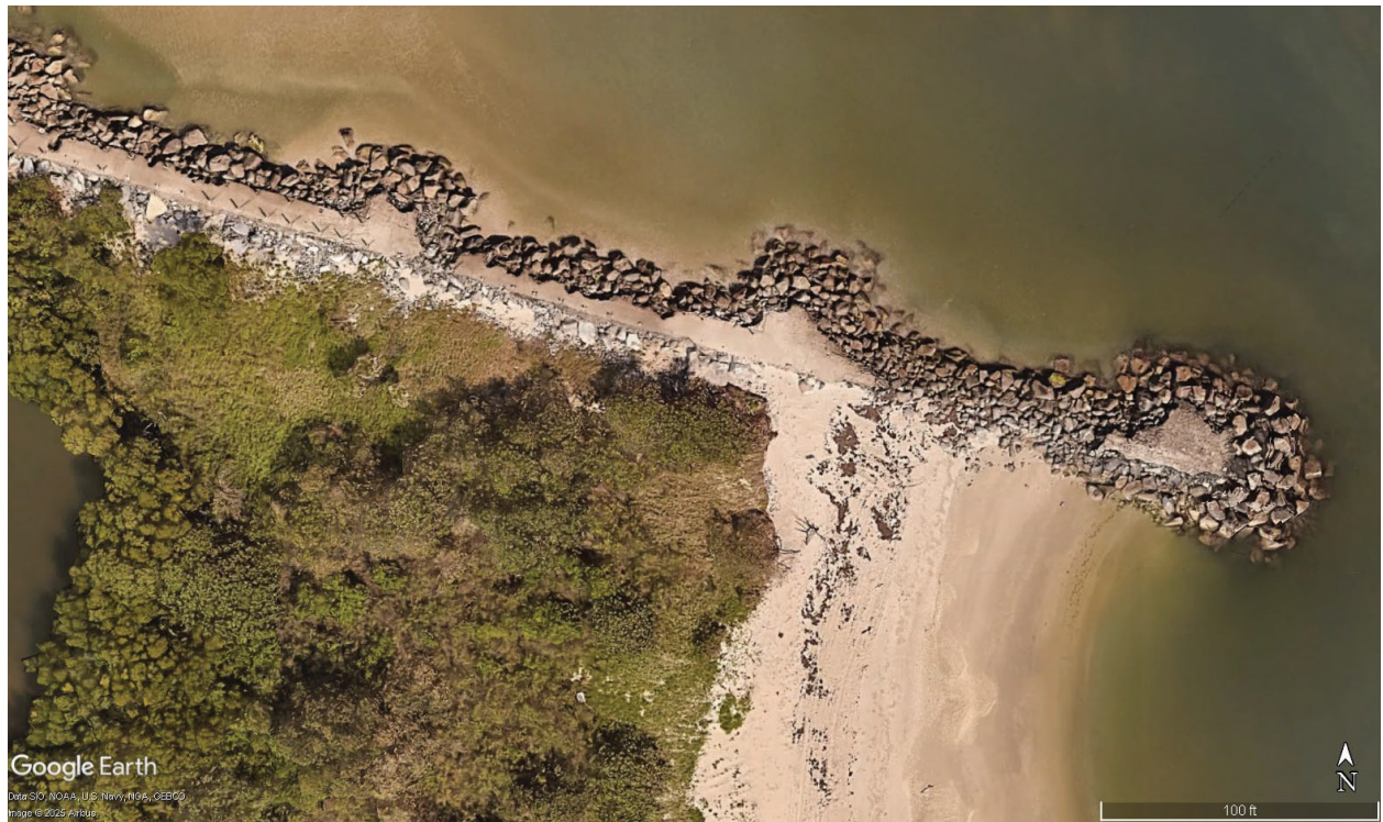
Figure 2: Close up view of the St. Lucie South Jetty Head
