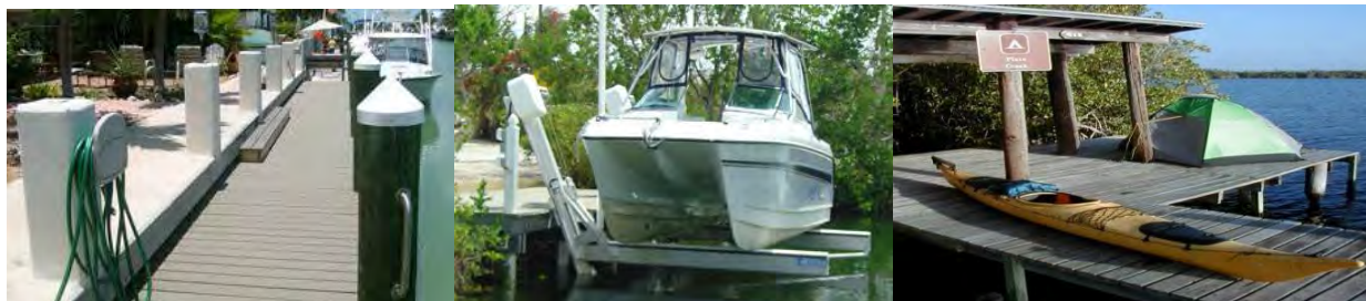
Figure 4. Example of a marginal dock on the left, boatlift with I-beam in the middle, and a chickee on the right. (The left and middle photos were provided by the Florida Marine Contractors Association and right photo from www.cnn.com .)
