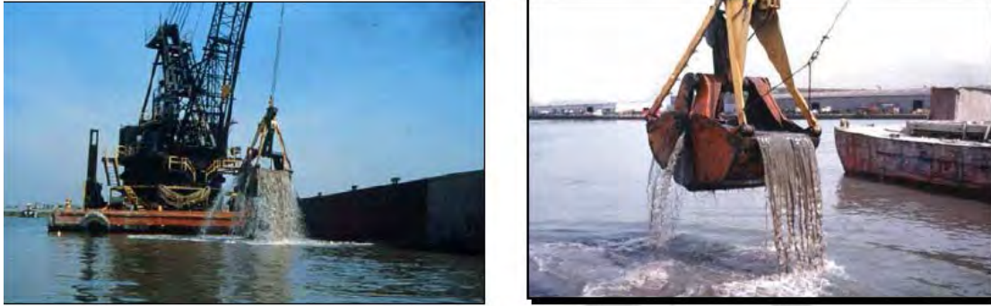
Figure 5. Mechanical dredge (clamshell bucket and barge)
