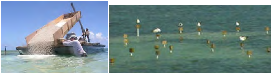
Figure 13. The left image is the placement of sediment to return a blowhole to pre-injury elevation. The image on the right shows bird stakes placed in a restoration area. (Both images are from www.darrp.noaa.gov .)
