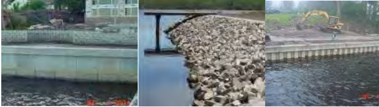
Figure 2. Example images of shoreline armoring and stabilization. The left image is a concrete slab seawall, middle is a riprap shoreline, and the right is a vinyl seawall. (Images provided by the Florida Marine Contractors Association)
