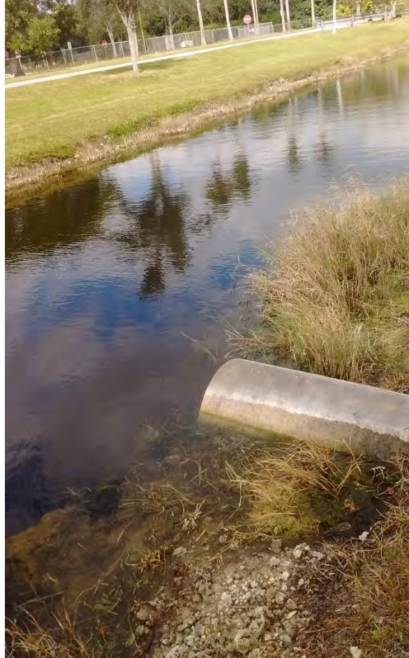
Photo 7: Culvert outfall from wetland in S-35 canal (northwest corner of property)
