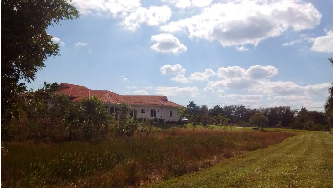
Photo 8: Western side of wetland and western edge of property (lawn) looking south. "Island 2" on left side of photo. "Island 3" non-existent.
