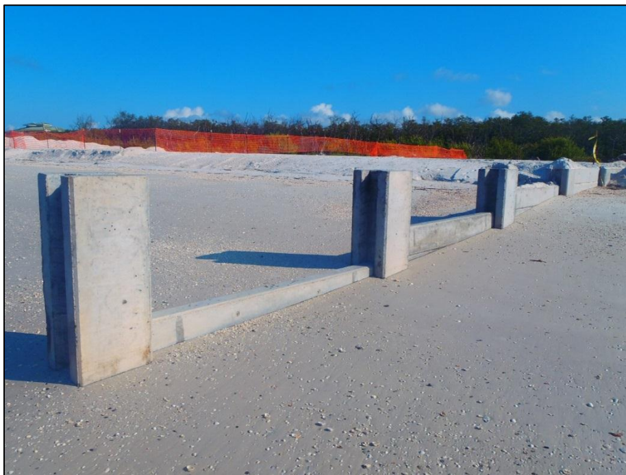
Figure 2-1 . Shoreward view of a concrete king pile and panel groin.
