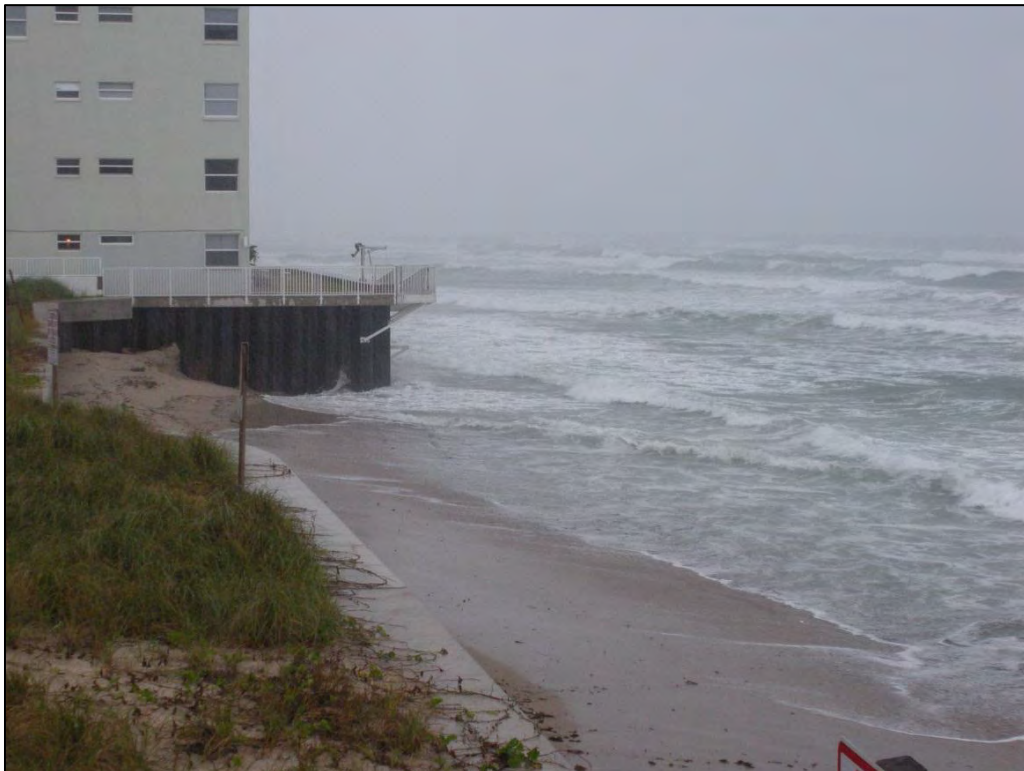
Figure 4-3. Impacts of Hurricane Sandy near R-137, Town of South Palm Beach (October 26, 2012).
