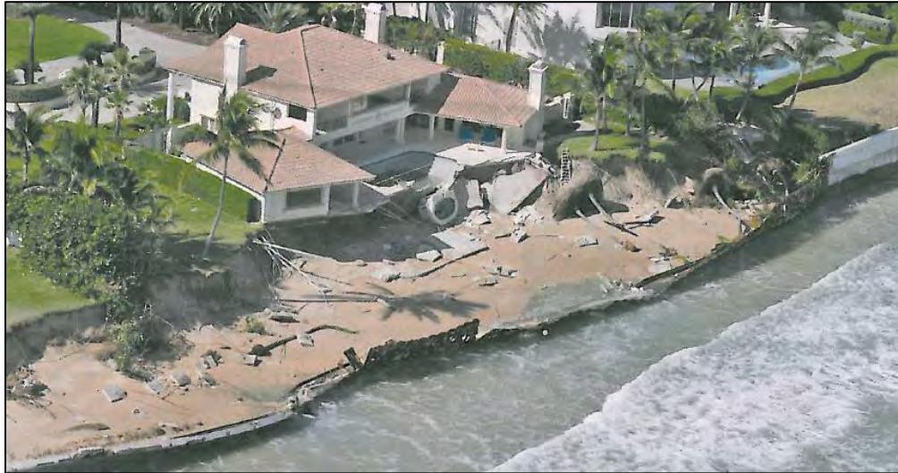
Figure 4-4. Failure of seawall in Manalapan after Hurricane Sandy (1 mile south of the Project Area, R-143.5) (Coastal Star, 2013).
