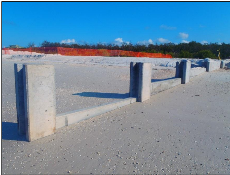
Photograph 2-1. Shoreward view of a concrete king pile and panel groin.
