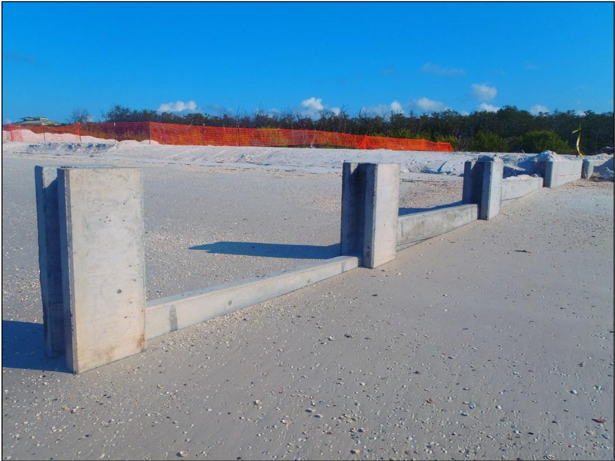
Photograph 6-1. Shoreward view of a concrete king pile and panel groin.
