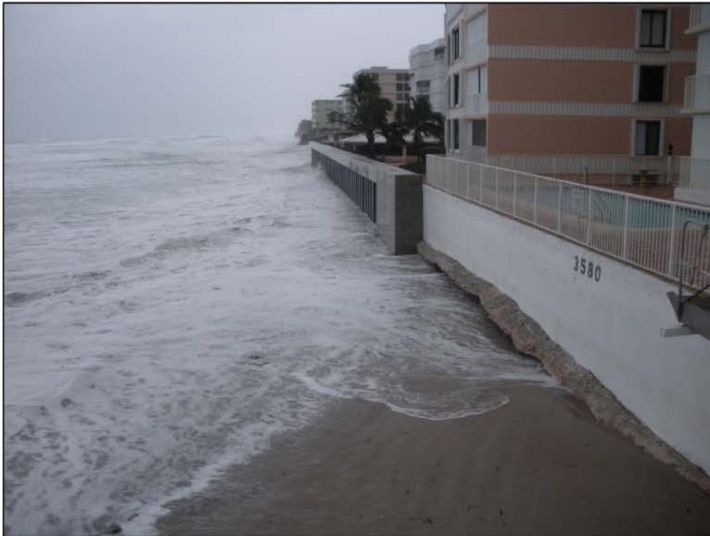
Figure 4-2. Impacts of Hurricane Sandy near R-136, Town of South Palm Beach (October 26, 2012).
