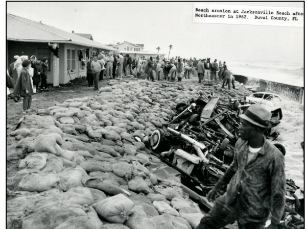
Jacksonville Beach erosion 1962.
