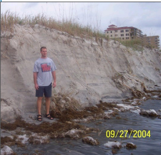
Erosion along Jacksonville Beach.
