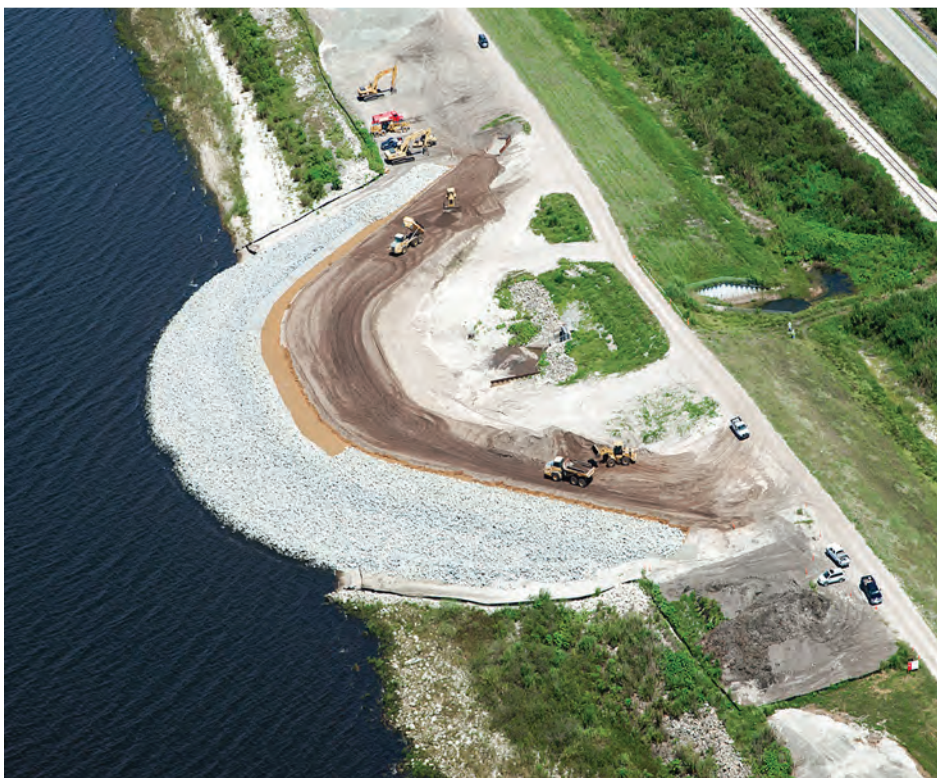
A temporary dam is constructed in advance of the removal of Culvert #14 near Port Mayaca. The culvert was removed in the fall of 2011. (Photo courtesy of Optimum Services, Inc)
