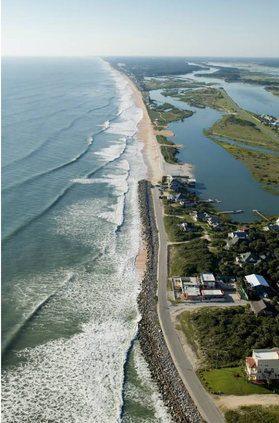
Figure 2-4. Summer Haven reach viewed from northern end. Granite revetment protects paved section of Old SR A1A.
