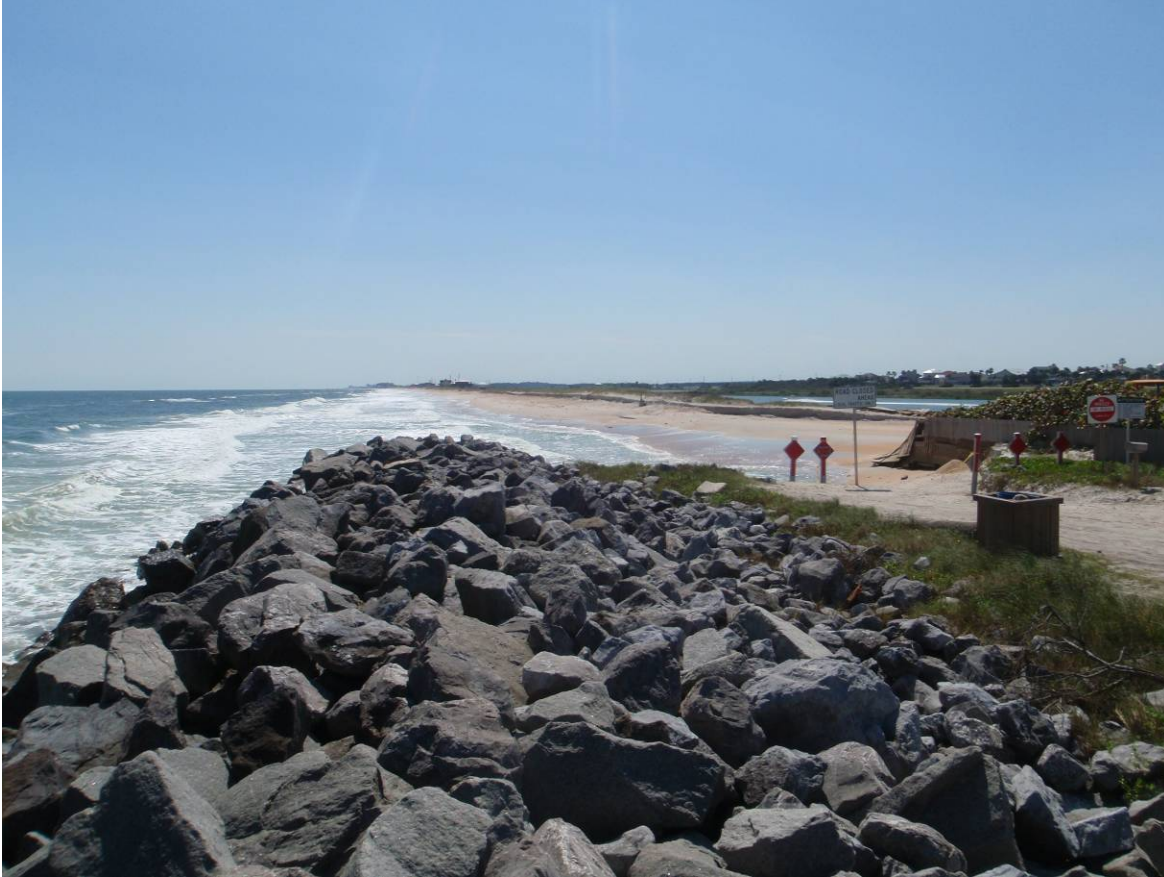
Figure 2-7. Looking south along the Summer Haven reach (around R198). Granite revetment fronts paved remnant of Old SR A1A. The breach at R200 is shown in the middle of the picture, just beyond the “Road Closed” sign.
