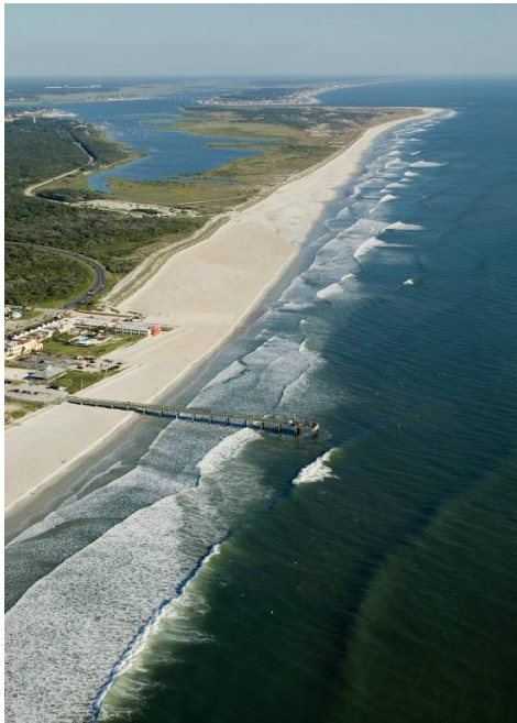
St. Augustine Beach – constructed
