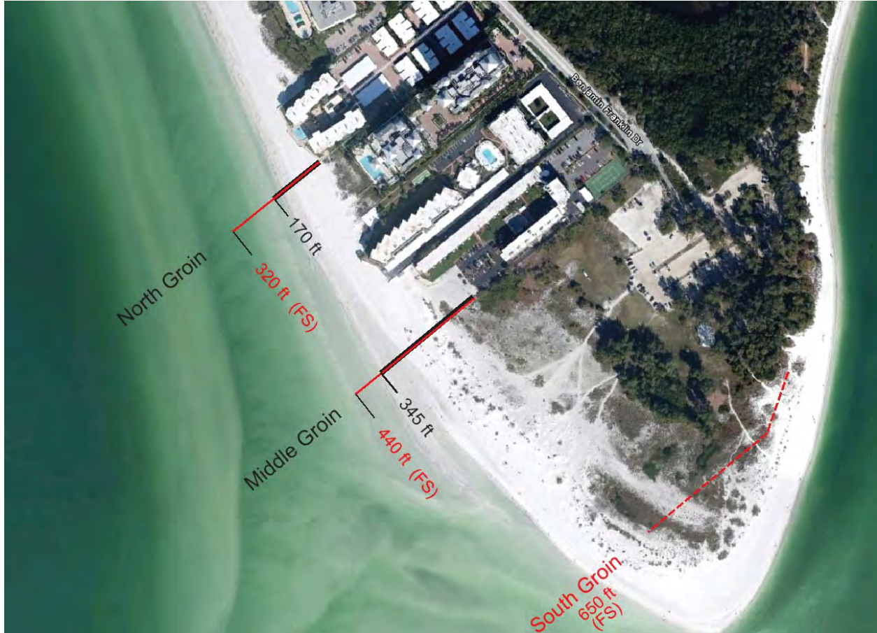
Figure 3. South Lido Key groin field. Recommended structure lengths are taken from the Feasibility Study (FS) and the 2014 reanalysis of the structures.
