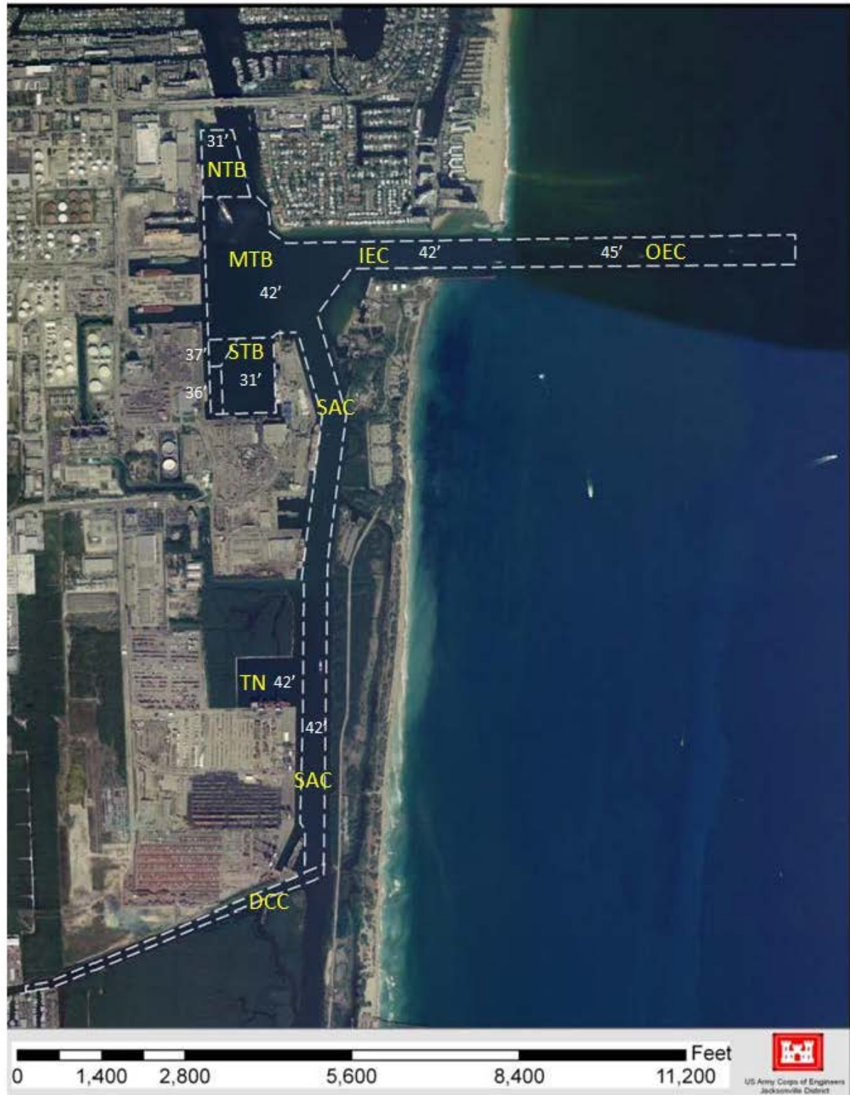
Figure 10. Existing Channel Components
