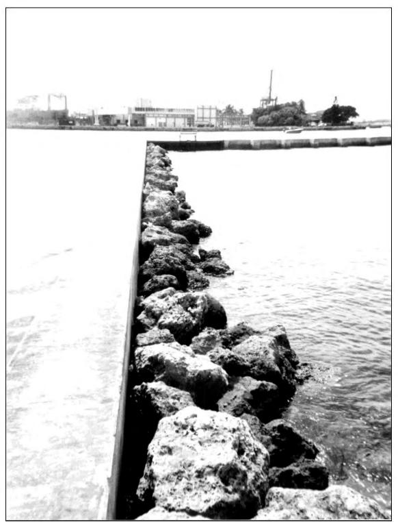
Figure 8. Example of Rubble Wave Absorber at USCG Fort Lauderdale (South Bulkhead)
