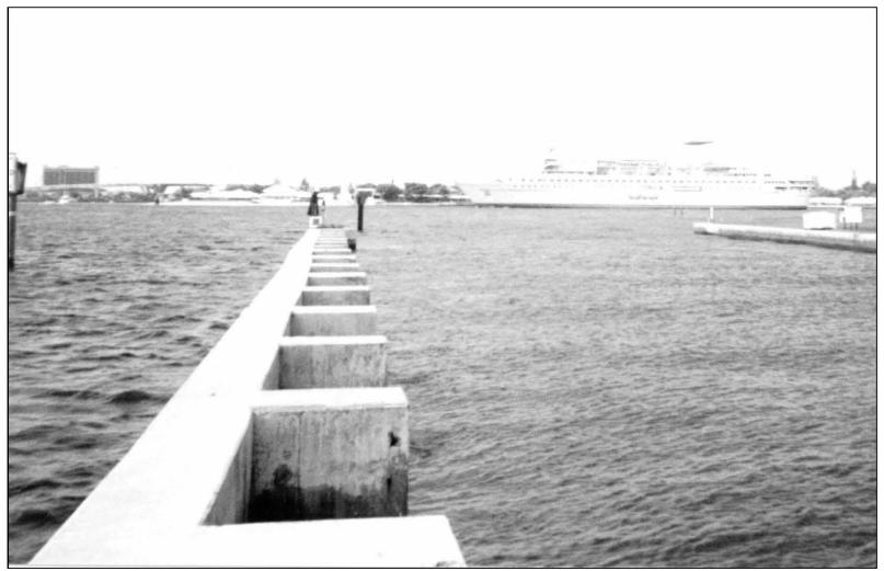
Figure 7. Example of Wave Damping Bulkhead at USCG Fort Lauderdale (Entrance Channel Bulkhead)
