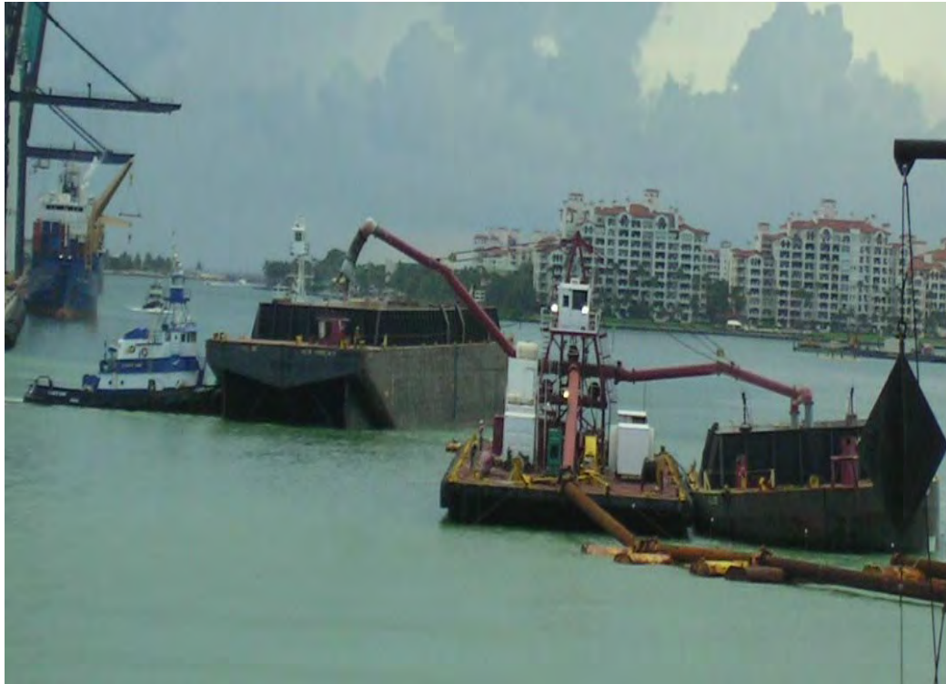
Figure 11. Loading two scows using a "spider barge."
