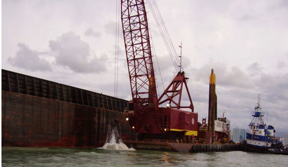
Figure 10. Loading a split-hull barge using a clamshell dredge.
