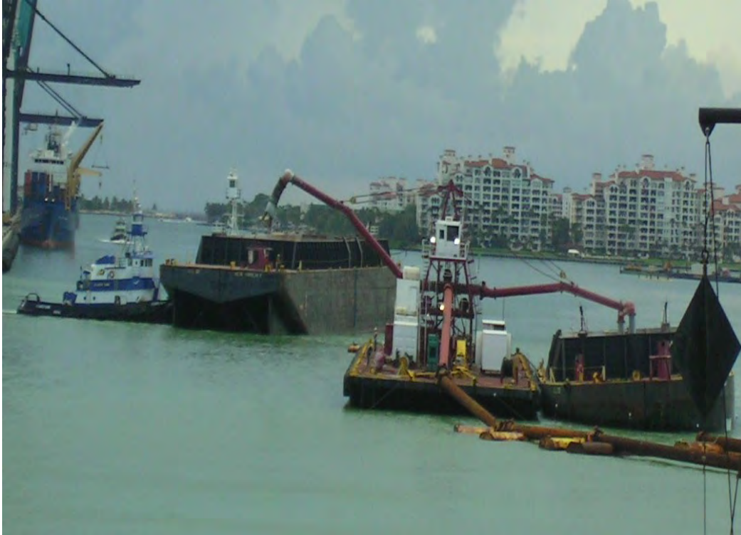
Figure 11. Loading two scows using a "spider barge."
