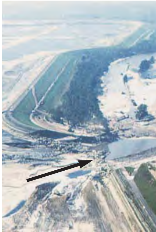
Breach of Florida Power and Light Cooling Reservoir, 1979. Failed due to piping of material from the foundation of the dike.
