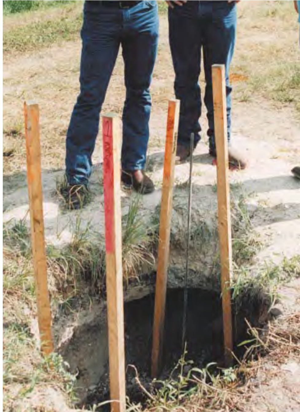
Sinkhole on levee crest at Lake Harbor site.
