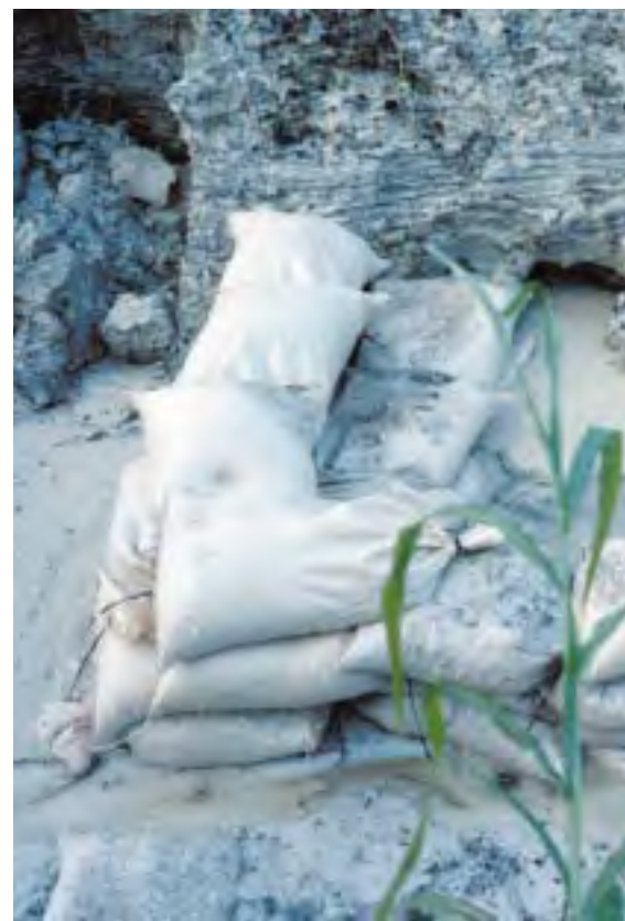
Sandbagging and piping at Lake Harbor showing mound of piped material that is flowing from the dike.
