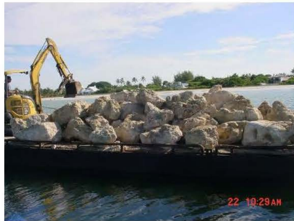
Unloading Operations of Reef Material
