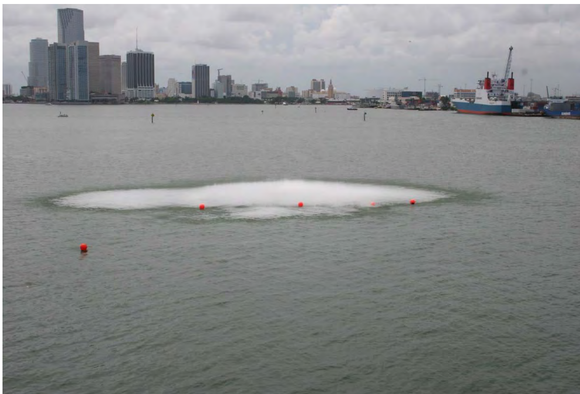
Figure 7 Confined Blast of 3,000 Pounds of Explosives
