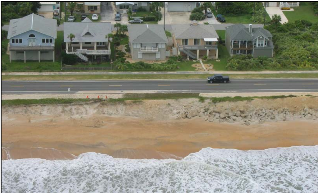
Figure 2-6: Looking west along SR A1A near R-68 on 23 August 2008, after Tropical Storm Fay. The rocks on the right side of the image were placed by FDOT as an emergency measure to protect SR A1A from being undermined by waves. Also, the sand on the road is a result of a complete wash over during the storm.
