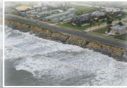
Flagler Beach erosion threatening homes, businesses, and State Road A1A; failing revetment
