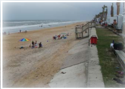
Beverly Beach erosion threatening oceanfront homes and State Road A1A
