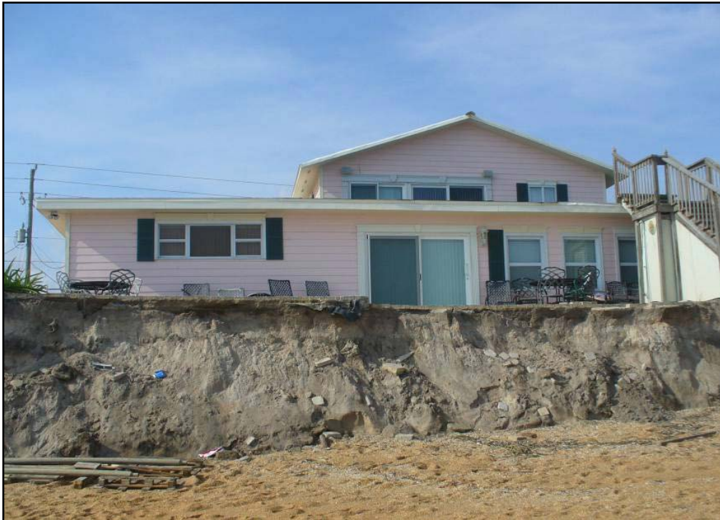
Figure 2-4: Beach erosion in Painters Hill following the December 2007 storm event.
