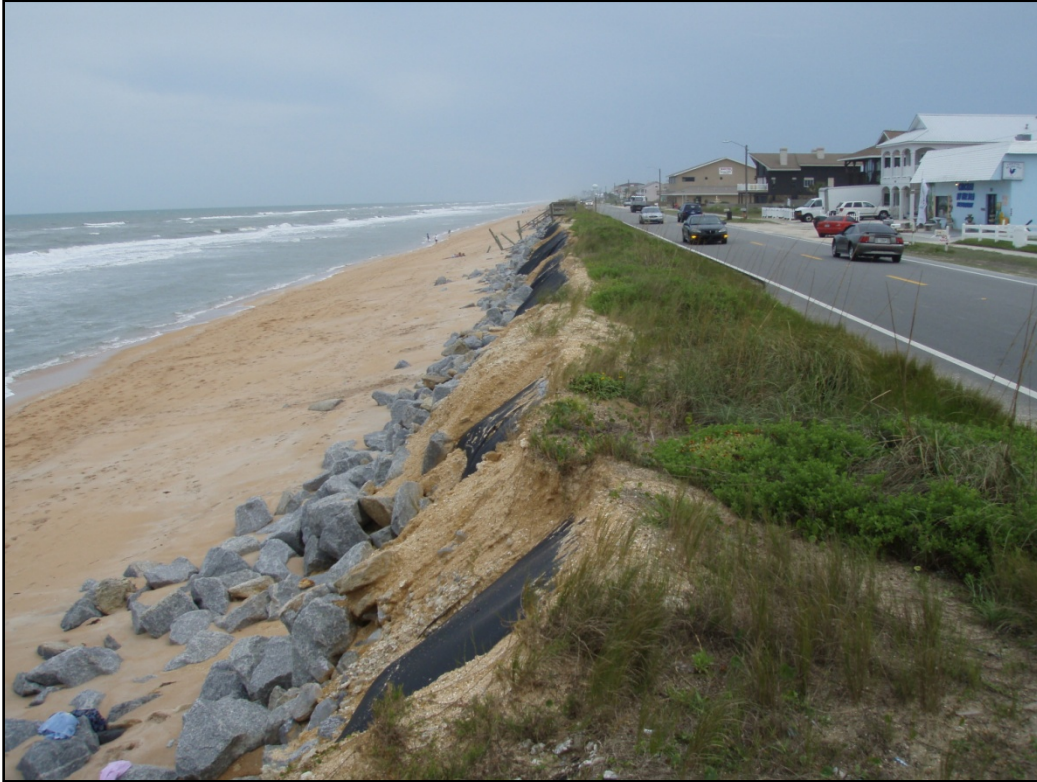
Figure 2-8: Looking south from 19 th Street South in Flagler Beach on 24 May 2009. This image was taken during low tide and the distance between A1A and the waterline was measured as approximately 75 feet. Notice the failing revetment and visible geotextile fabric which is meant to line the underside of the revetment.
