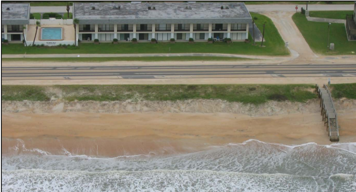
Figure 2- 5: State Road A1A at the border of the Beverly Beach and Flagler Beach reaches immediately after Tropical Storm Fay in August 2008. Sand has been washed over the dune and deposited on the road.
