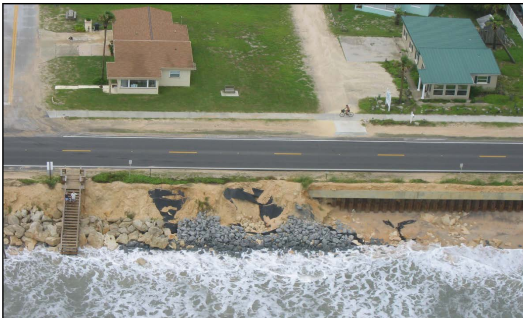
Figure 2-7: Aging seawall and revetment protecting SR A1A from the eroding shoreline in Flagler Beach.
