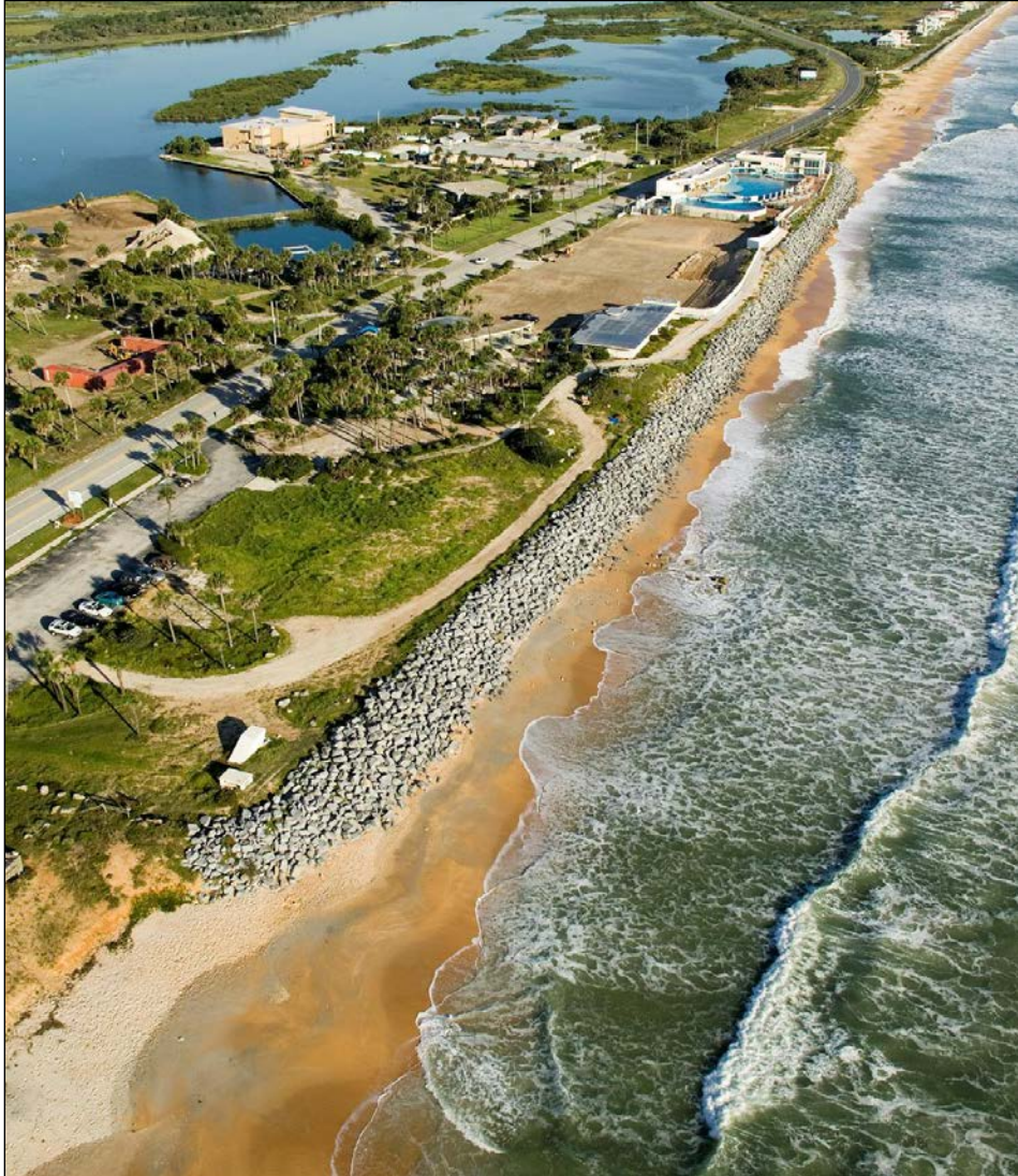
Figure 2-2: The 1,350-foot long granite revetment and one partially buried coquina groin in the Marineland study reach. Three more coquina groins exist to the south of the revetment.
