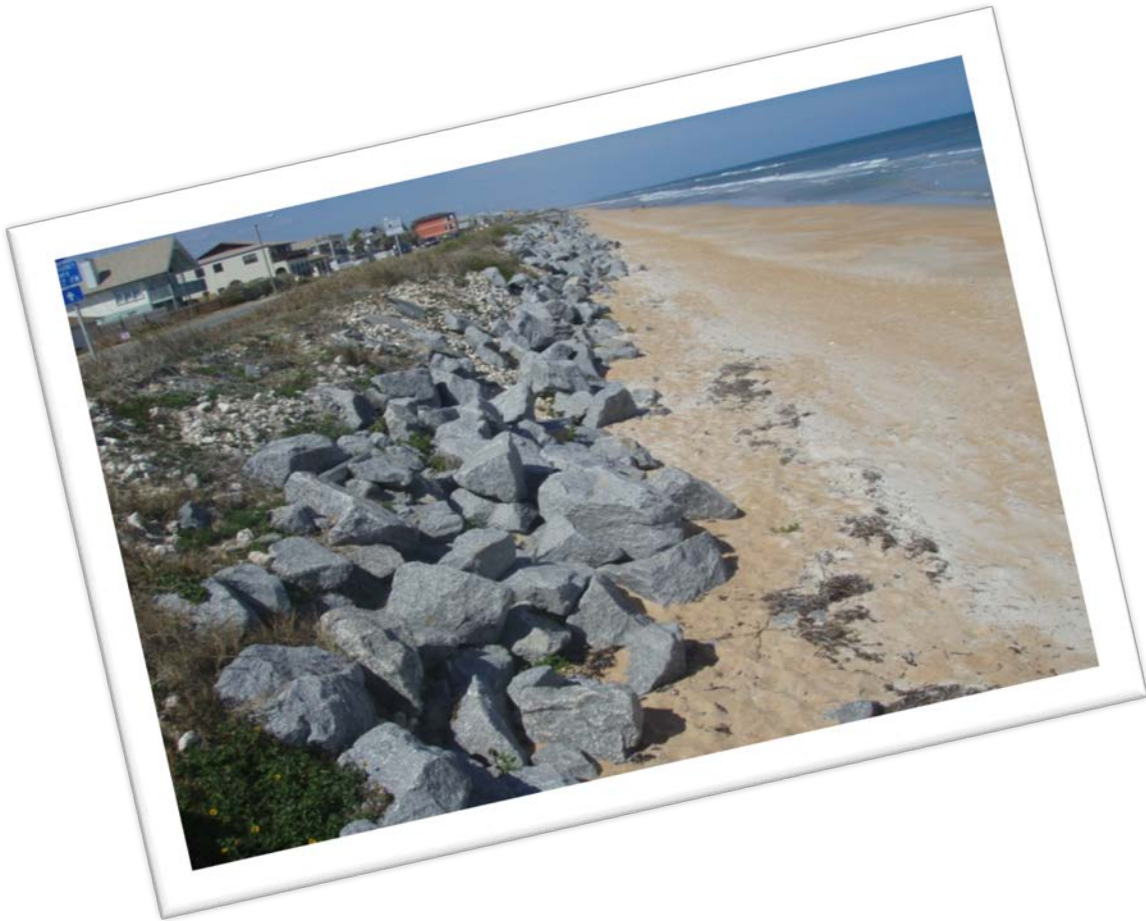
Figure 2-1: Revetment protecting SR-A1A in Flagler Beach
