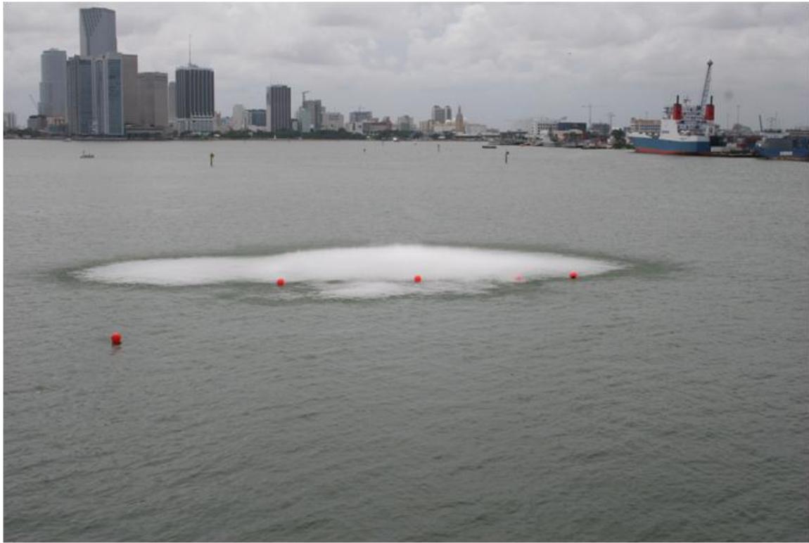
FIGURE 30: CONFINED BLAST OF 3,000 POUNDS OF EXPLOSIVES
