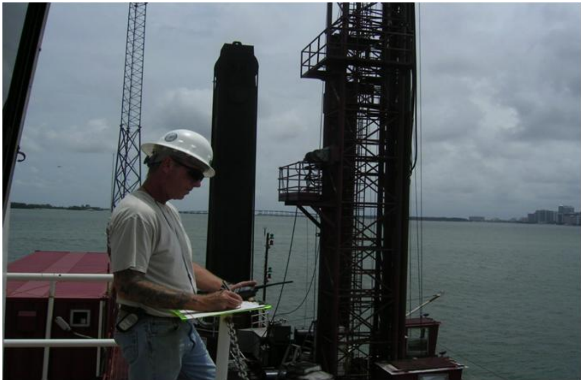
FIGURE 35: OBSERVER ON DRILL BARGE
