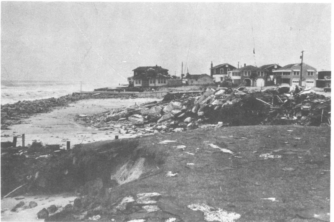
NEPTUNE BEACH, FLORIDA AFTER HURRICANE DORA September 1964
