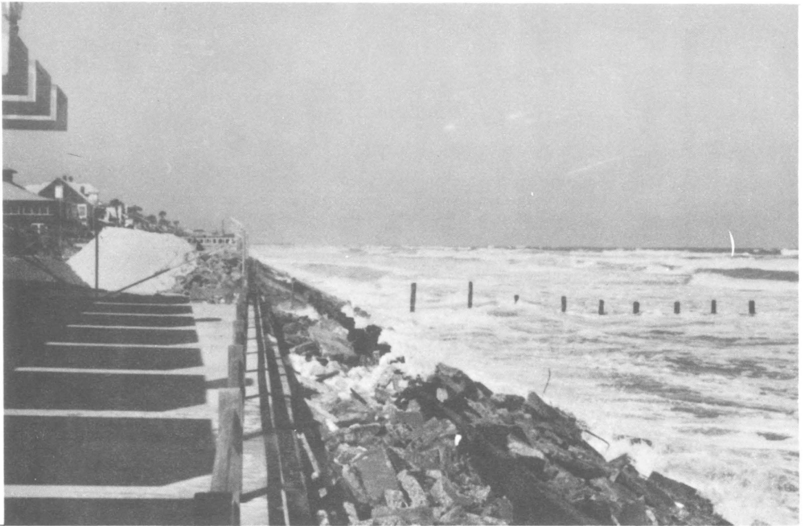
NORTH OF ATLANTIC BOULEVARD ATLANTIC BEACH, FLORIDA
