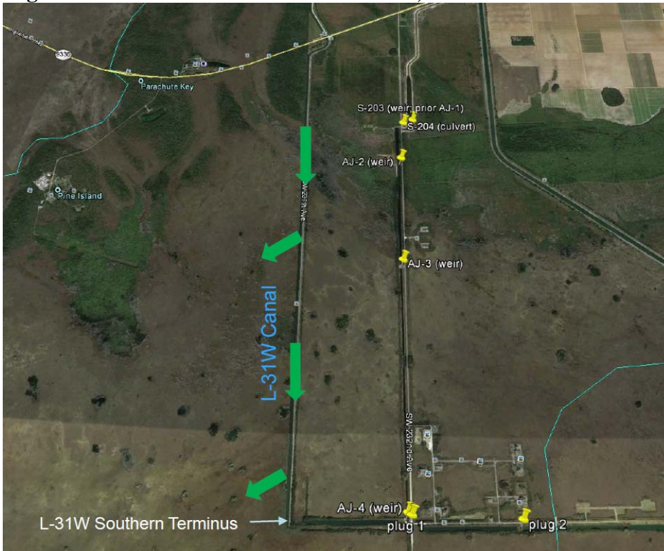
Figure 12. Southern Reach of L-31W Canal, South of State Road 9336
