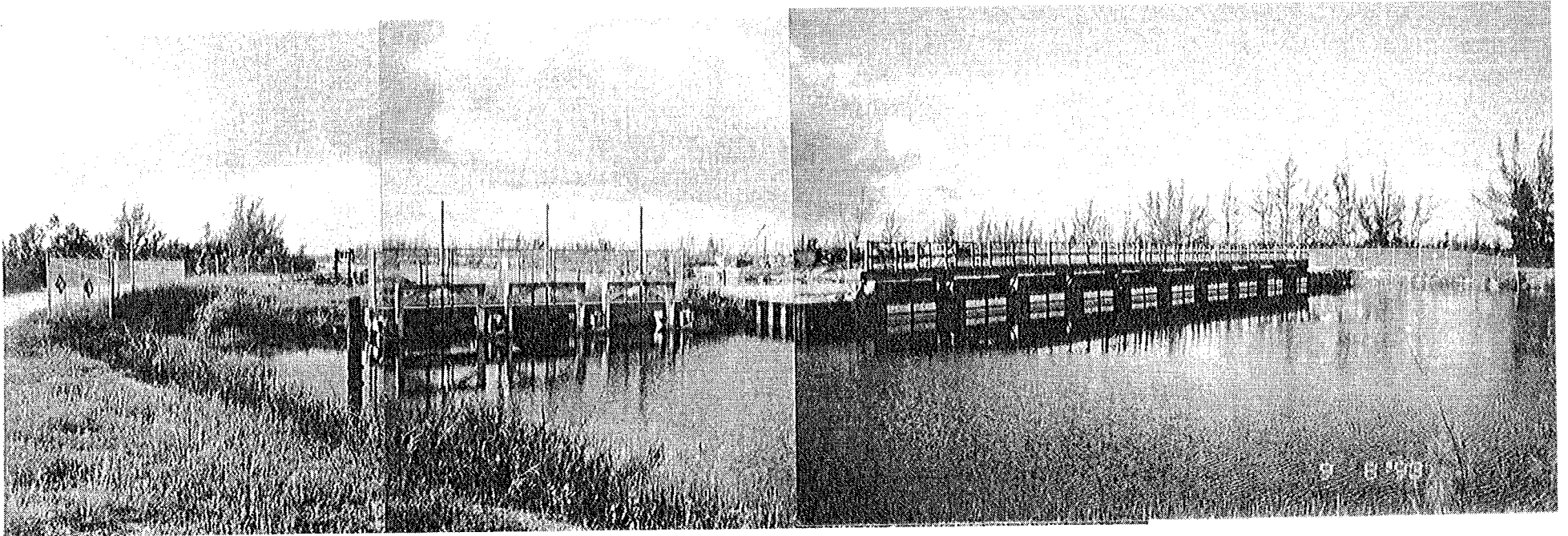
PHOTO A-14. LOOKING AT THE UPSTREAM SIDE OF S-197, THE THREE ORIGINAL CULVERTS AT LEFT, AND THE TEN ADDITIONAL INSTALLED BY THE LOCAL SPONSOR AT RIGHT.
