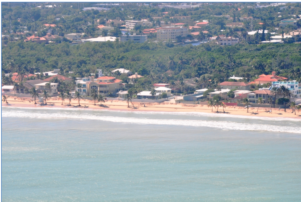
Figure 4 - Area of damage to S.R. A1A. Sand scraped from roadway as a result of overwash is placed along seaward side of road). Photo taken at NE 16th Ct, Ft. Lauderdale.
