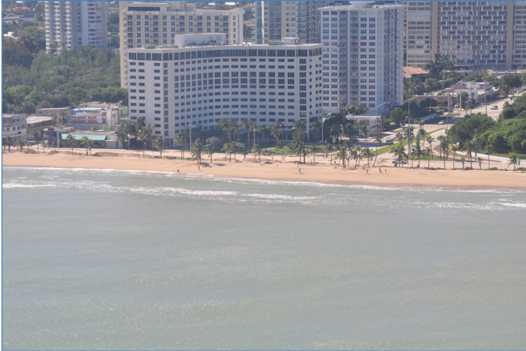
Figure 5 - Sand scraped off of adjacent roadways as a result of overwash (placed as a dune-line along seaward side of A1A). Photo taken at E. Sunrise Blvd, Ft. Lauderdale
