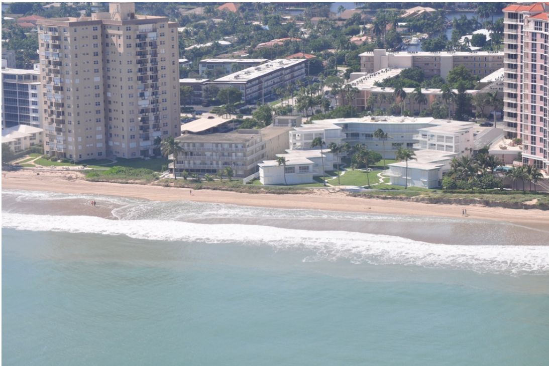
Figure 2 - Loss of berm width and height, scarping into dune line. Photo taken at Bel Aire Drive, northern Lauderdale-by-the-Sea
