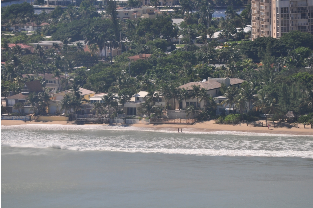
Figure 3 - Loss of berm width and elevation. Significant erosion in front of seawalls, some houses within 30 feet of waterline. Photo of NE 28th St. Fort Lauderdale
