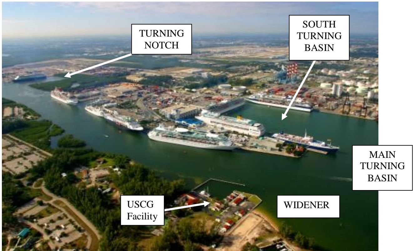
Figure 24: Northern Channel Improvement Areas Looking Southwest
