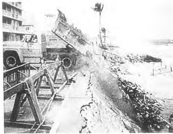
Figure 7. Emergency dumping of riprap in the late 1960s to protect a coastal highway at Delray Beach (Courtesy of Coastal Planning and Engineering, Inc.).
