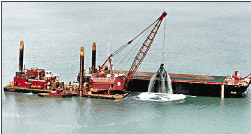
Figure 8: Mechanical dredging; clamshell dredge with scow. (Photo: Great Lakes Dredge & Dock Co.)
