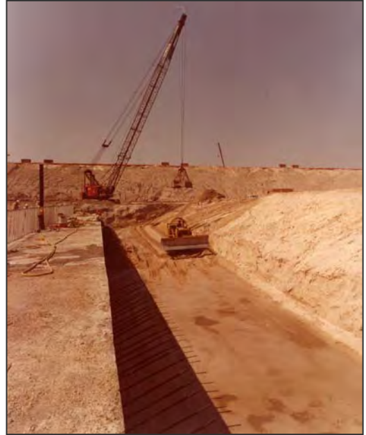
Figure 4: Concrete sill under construction – note extensive rebar.
