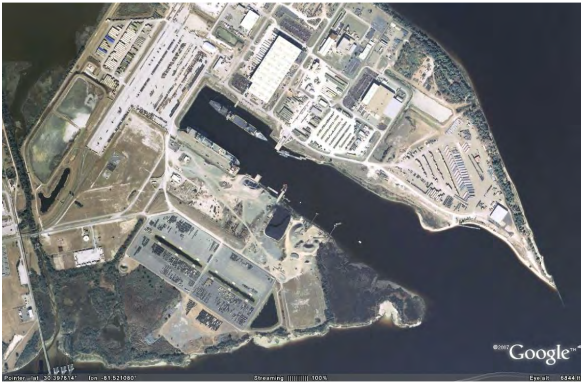
Figure 3 - Close up of MSCF-BI slipway
