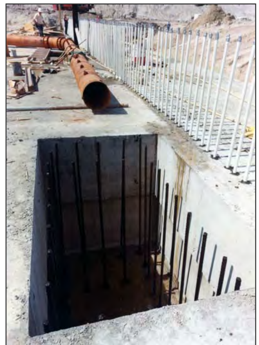
Figure 6: Rebar reinforcement of – concrete sill.
