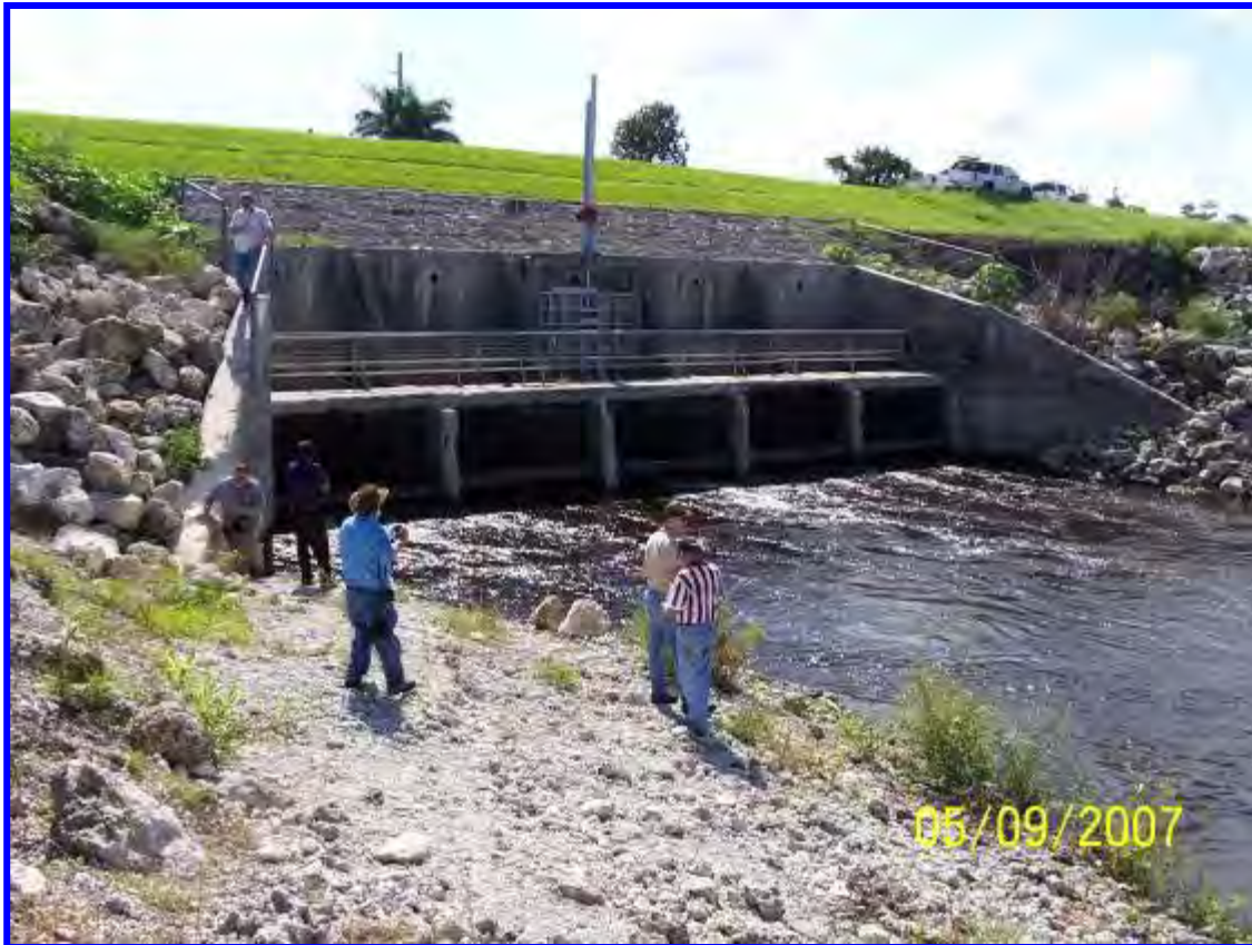
Figure 3. Culvert 10A - Concrete Wing Wall Heavily Pitted with Exposed Rebar
