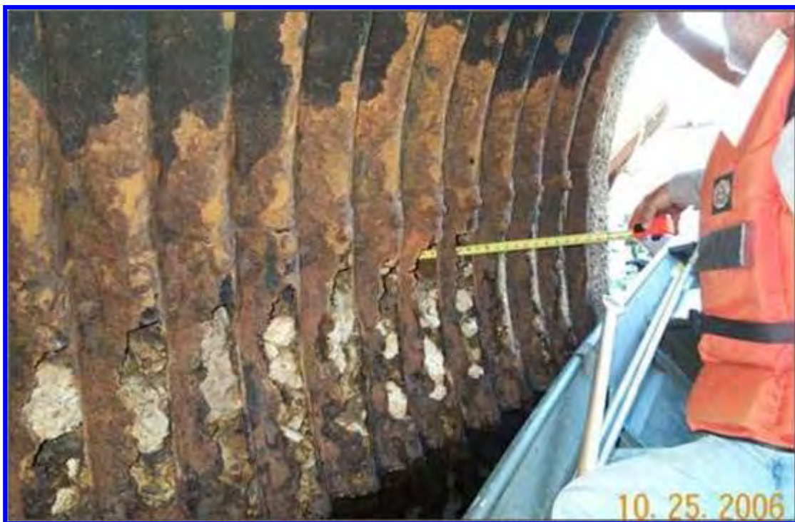
Figure 4. Culvert FC-1 – Corrosion through Barrel, Exposing Cobble Layer of Embankment
