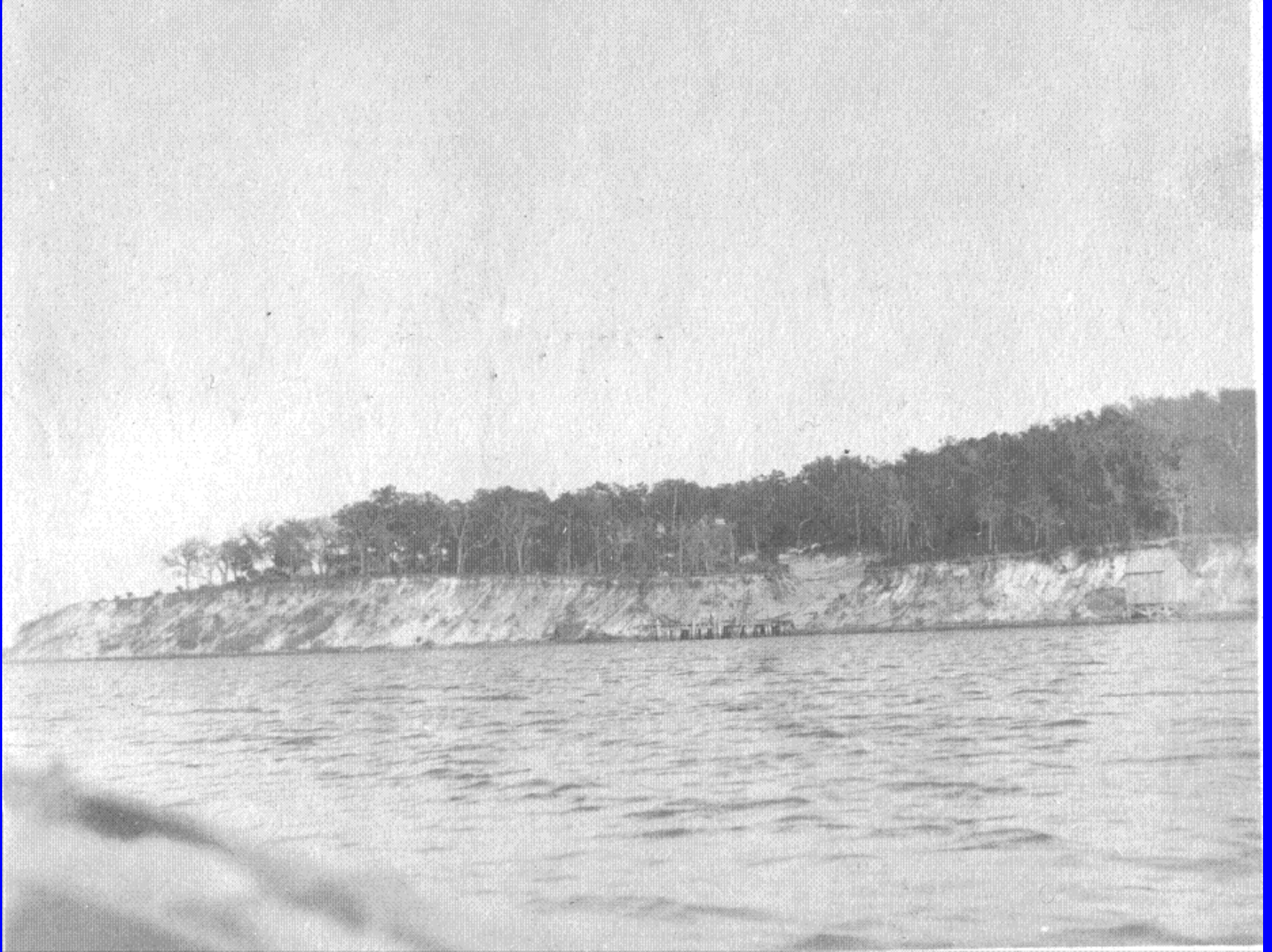
St. Johns Bluff c-1900 shows dock and cut in bank for construction of Spanish/American War Batteries. Possible mine field terminal on right
