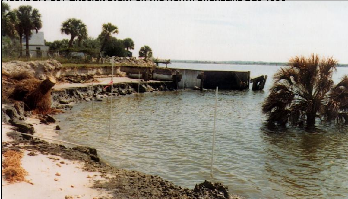
FIGURE 2: POST-EROSION EVENT ON THE NORTH SHORELINE DEC 1990
