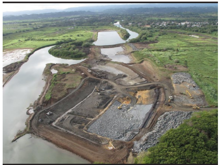
This recent aerial shows construction progress on the Río de La Plata project. The river flows by the municipality of Dorado, about 15 miles west of San Juan on the northern coast of Puerto Rico. Looking upstream, the photo shows channel excavation and placement of stone revetment (right), while the river flows through a temporary diversion channel to the left. The revetment will slow the velocity of storm water coming from the mountains upstream and prevent erosion of the banks. (PHOTO COURTESY OF CONSTRUCCIONES JOSÉ CARRO)
