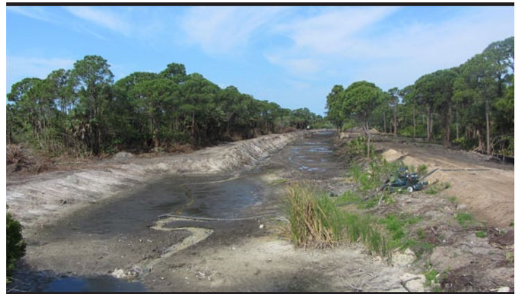
A current view of the filter marsh, in which invasive vegetation has been removed. A new weir structure will be constructed, where flows will outfall into an existing slough system that discharges into the east branch of Coral Creek. Wood Storks and Roseate Spoonbills have already been observed feeding in the marsh as it was pumped down. (PHOTO BY STEPHANIE POWERS, SWFWMD)
