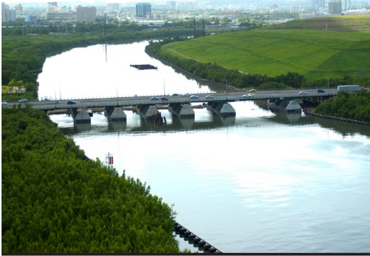
Looking upstream to its source in the central mountains, the Río Puerto Nuevo basin drains 24 square miles of metropolitan San Juan, 75 percent of which is highly developed with a population of 250,000. The plan of improvements includes channels, high velocity channels, debris basins and modifications to bridges, in an effort to protect the population against a 100-year flood. (USACE PHOTO)
