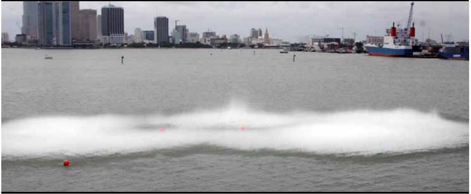
Confined blasting method, using 3,000 pounds of explosives to crack rock beneath the water's surface in Miami Harbor. (PHOTO BY TERRI JORDAN-SELLERS).
