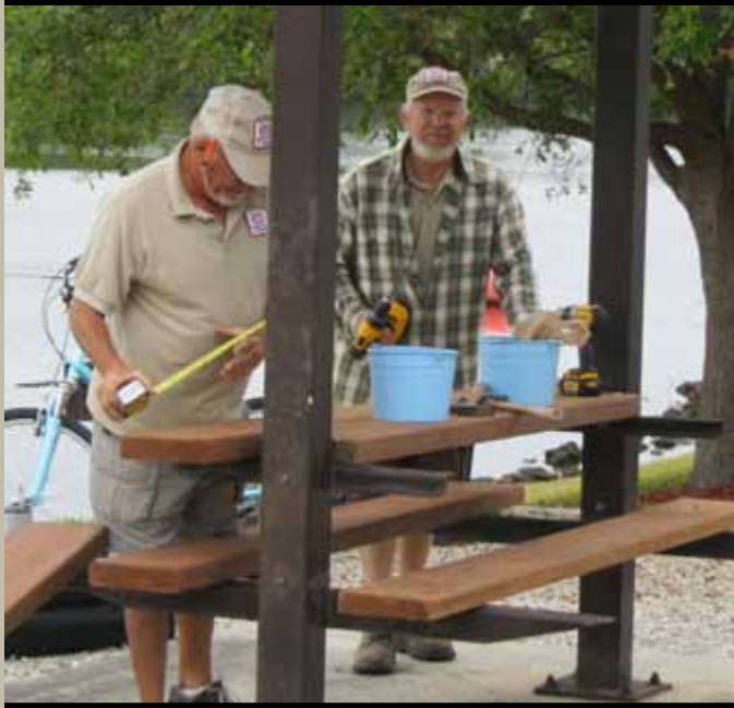
W.P. Franklin and Lock volunteers measure twice and cut once when replacing re-planed boards in shelters. (PHOTO COURTESY OF PHIL HART)
