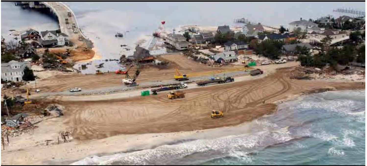
The U.S. Army Corps of Engineers worked rapidly to repair a levee breach caused by Hurricane Sandy in Mantoloking, N.J. The breach occurred at the end of the only bridge onto the barrier island, effectively cutting it off from the rest of the state. At the peak of the response effort, the Corps had nearly 4,000 employees from across the nation engaged in more than 38 FEMA mission assignments, exceeding a total of $134 million. (PHOTO BY MARY MARKOS, ST. LOUIS DISTRICT)
