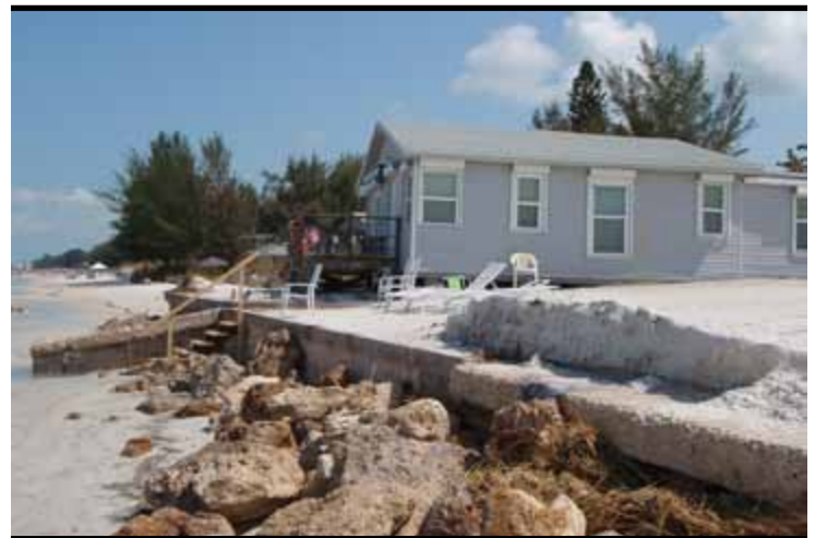
Significant beach erosion in Manatee County, resulting from Tropical Storm Debby. (PHOTO COURTESY MARTY DURKIN)
