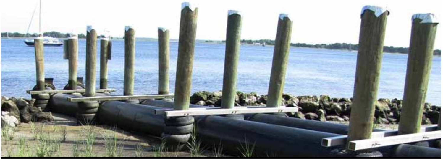
Buck Island Cell A weirs, designed by Coraggio Maglio, won him the 2012 USACE Innovation of the Year Award. Once the design is fully vetted with other districts, it has the potential to revolutionize the way the Corps designs decanting systems. (PHOTO BY CORAGGIO MAGLIO)
