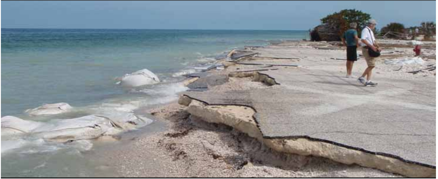
Local officials look at the remains of a parking lot in Pinellas County next to the Gulf of Mexico. Tropical Storm Debby caused significant beach erosion in six counties along the Gulf Coast. Jacksonville District dispatched a team to gather data as part of the formal damage assessment process. (PHOTO COURTESY MARTY DURKIN)
