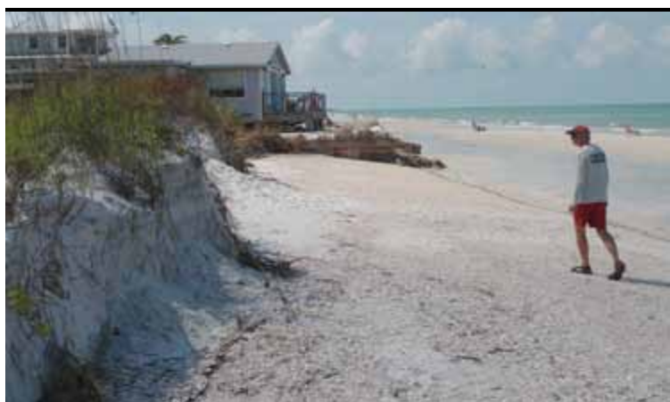
A local sponsor looks at beach erosion resulting from Tropical Storm Debby in Manatee County. Jacksonville District sent a team after the storm left the area to inspect damage and gather data to use in recovery programs administered by the Corps and FEMA. (PHOTO COURTESY MARTY DURKIN)
