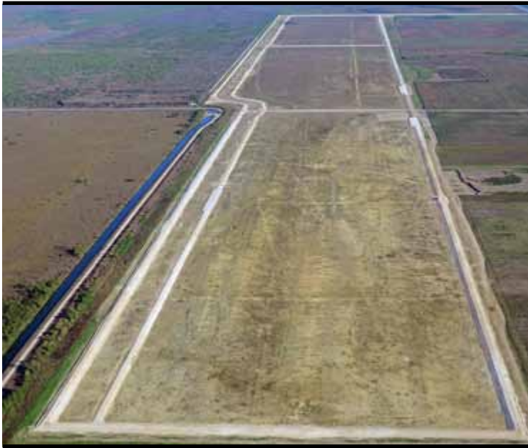
The 590-acre Frog Pond Detention Area, a component of the C-111 Spreader Canal Western Project, has three cells and three emergency spillways that are used to retain water in Everglades National Park by decreasing seepage to the east into the C-111 Canal. (PHOTO COURTESY SOUTH FLORIDA WATER MANAGEMENT DISTRICT)
