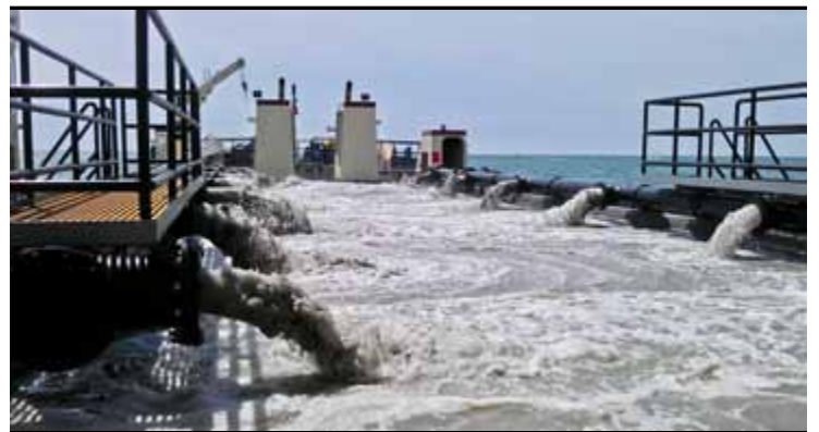
MURDEN begins dredging operations at Clearwater Pass. The hopper capacity is 512 cubic yards and disposes of the material via a split hull capability. (PHOTO BY JOSE BILBAO)
