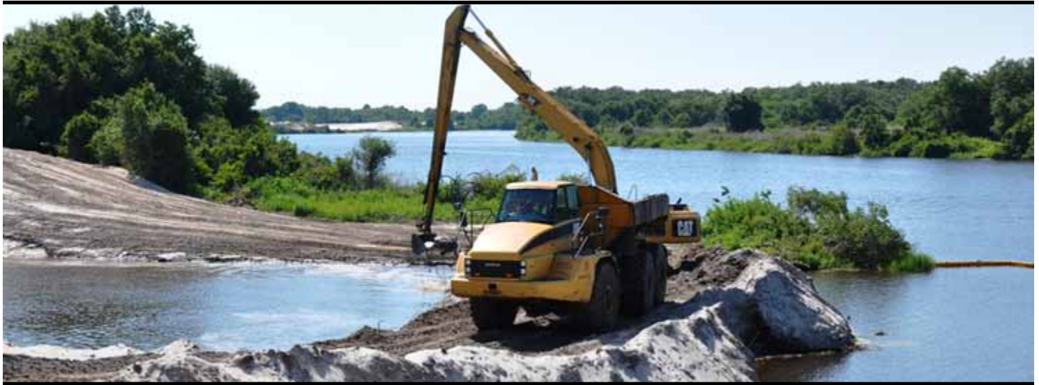
A large excavator removed the last earthen plug, connecting the historic channel to the channelized Kissimmee River.
