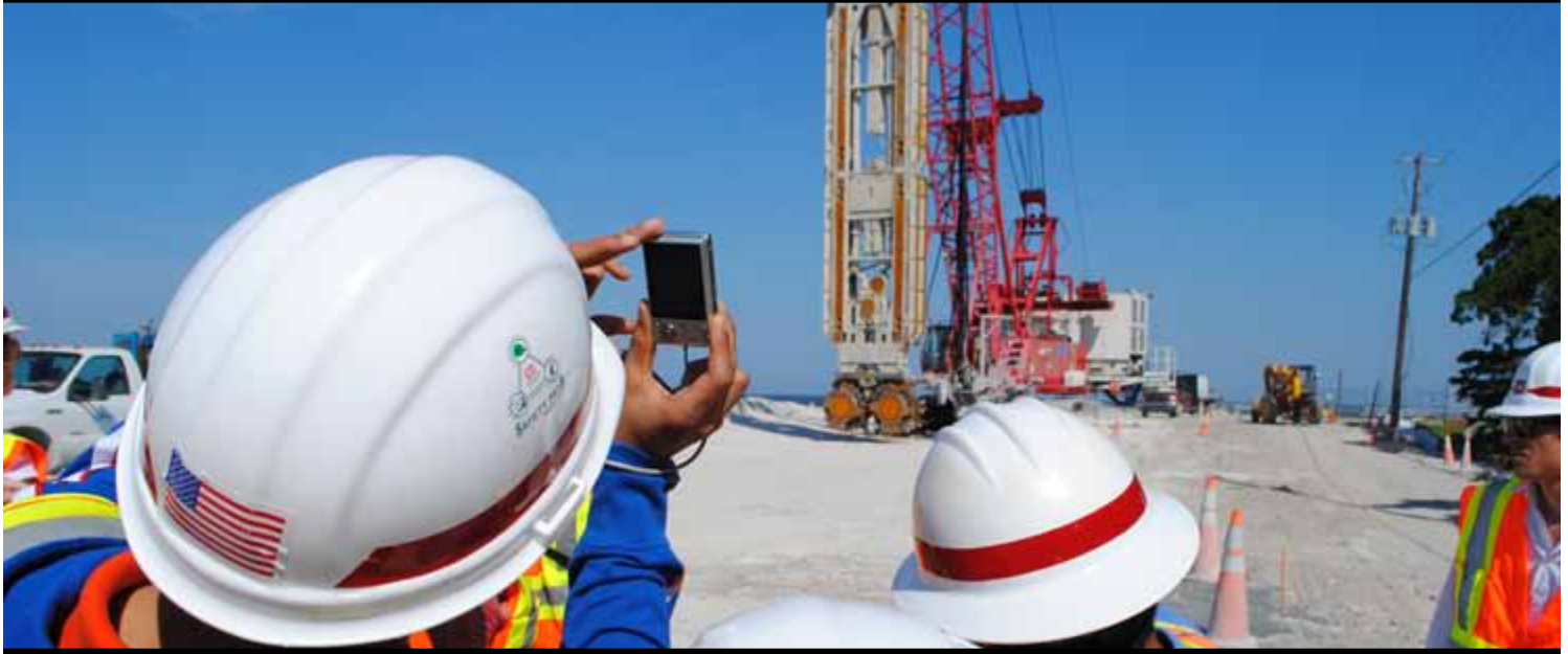
A student from UNESCO's Institute for Water Education photographs a "hydromill" attached to a crane at an HHD worksite near Port Mayaca.
