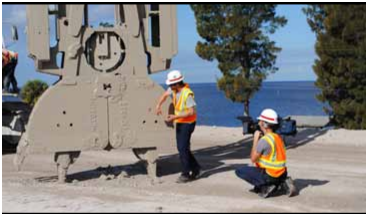
Don Wildman, host of The Travel Channel program "Off Limits," explains the workings of a "clamshell" while his cameraman rolls tape during shooting of rehabilitation activities at Herbert Hoover Dike in late January.
