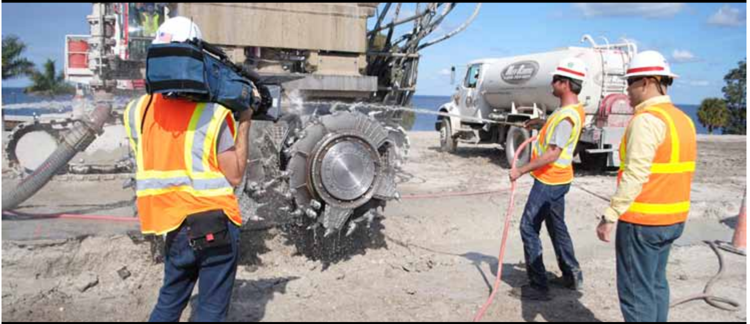
"Off Limits" program host Don Wildman of The Travel Channel assists with cleaning of the hydromill, used to install cutoff wall at Herbert Hoover Dike. Coaching him is Juan Sanchez-Bulted (right), civil engineer, Construction Division.
