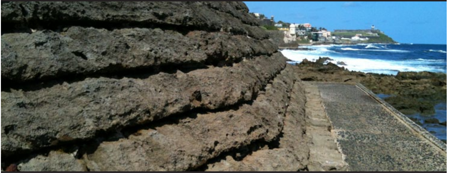
The excellent condition of a similar scour apron design constructed by the Corps in the late 1970s at the Devil's Sentry Box and La Perla was proof it should be used at Fort San Cristobal. (PHOTO BY JAIME CRUZ)
