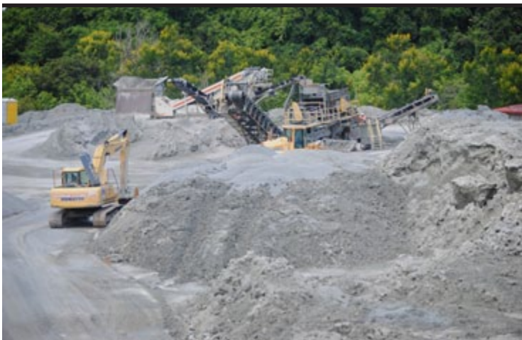
Left - Tons of sand and other aggregates are used in the construction of Portugues Dam. Crews constructed a complex mixing system on site to place the concrete into the dam. Right - Portugues Dam, June 2012. Pouring of the roller-compacted concrete (RCC) has been completed. Crews continue finishing work on the dam, to include placement of a "grout curtain" to prevent seepage beneath the dam. (PHOTOS BY JOHN CAMPBELL)
