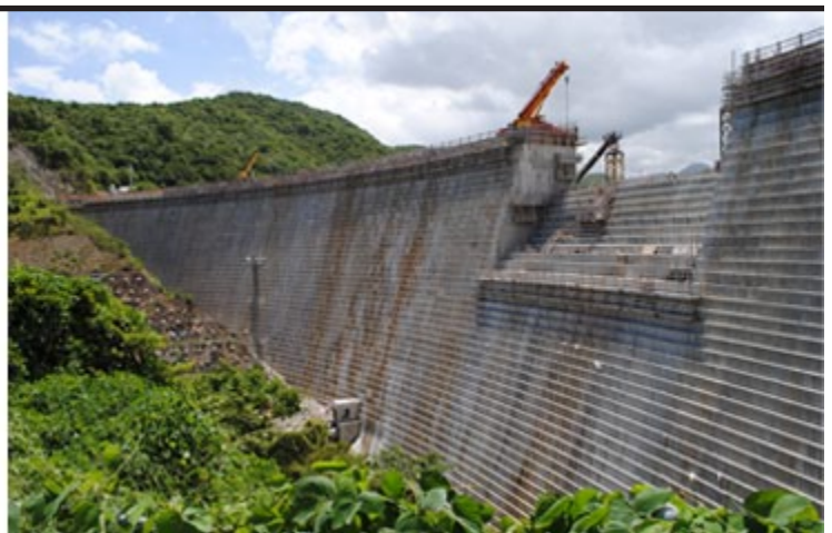
Left - Tons of sand and other aggregates are used in the construction of Portugues Dam. Crews constructed a complex mixing system on site to place the concrete into the dam. Right - Portugues Dam, June 2012. Pouring of the roller-compacted concrete (RCC) has been completed. Crews continue finishing work on the dam, to include placement of a "grout curtain" to prevent seepage beneath the dam. (PHOTOS BY JOHN CAMPBELL)
