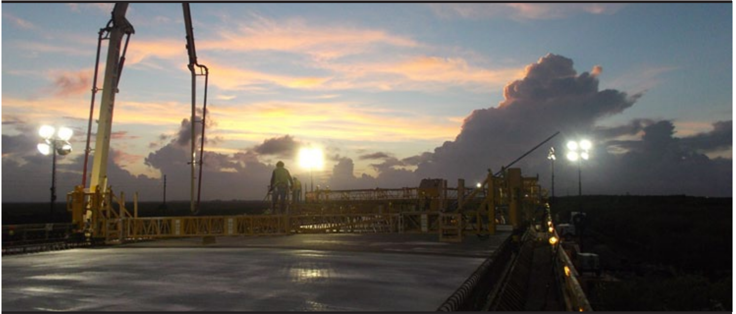
A major milestone for the Tamiami Trail Modifications project was reached shortly after midnight July 13 as the first concrete pour on the bridge deck was completed. (PHOTO BY RORY HIGHSTONE, KIEWIT CONSTRUCTION)
