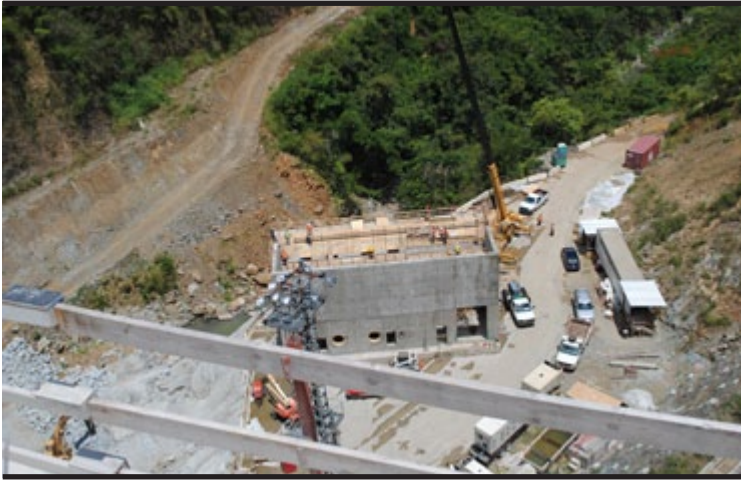
A view from the top of Portugues Dam looking at the valve house currently under construction. The dam is expected to be operational in the fall of 2013. (PHOTO BY JOHN CAMPBELL)
