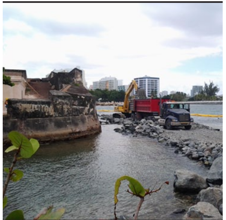
Armor stone is delivered to construct the revetment at Fort San Geronimo. (PHOTO BY JAIME CRUZ)
