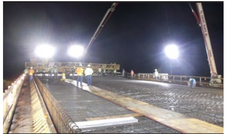
Jacksonville District employees and contractor, Kiewit Construction, work through the night to complete the first concrete pour on the bridge deck for the Tamiami Trail Modifications project. (PHOTO BY RORY HIGHSTONE, KIEWIT CONSTRUCTION)
