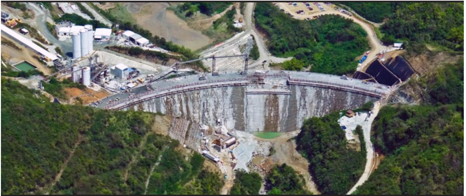
March 2012 aerial shot of Portugues Dam, with concrete construction still under way. (USACE PHOTO)
