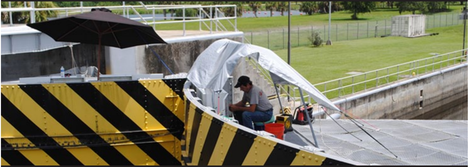
A contractor calibrates equipment for the Manatee Protection System, which was installed recently at the Moore Haven Lock. The lock resumed operations on July 14, about three weeks ahead of schedule. (USACE PHOTO)
